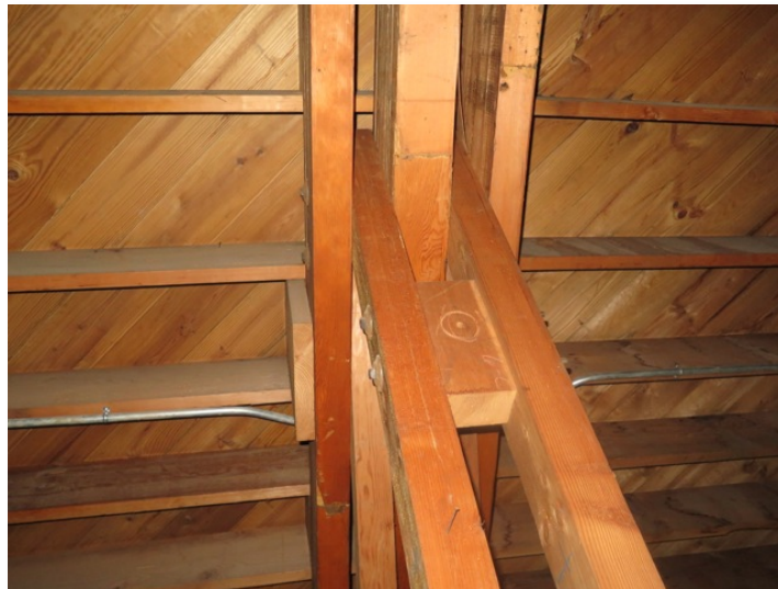
The wood component Bowstring roof trusses
