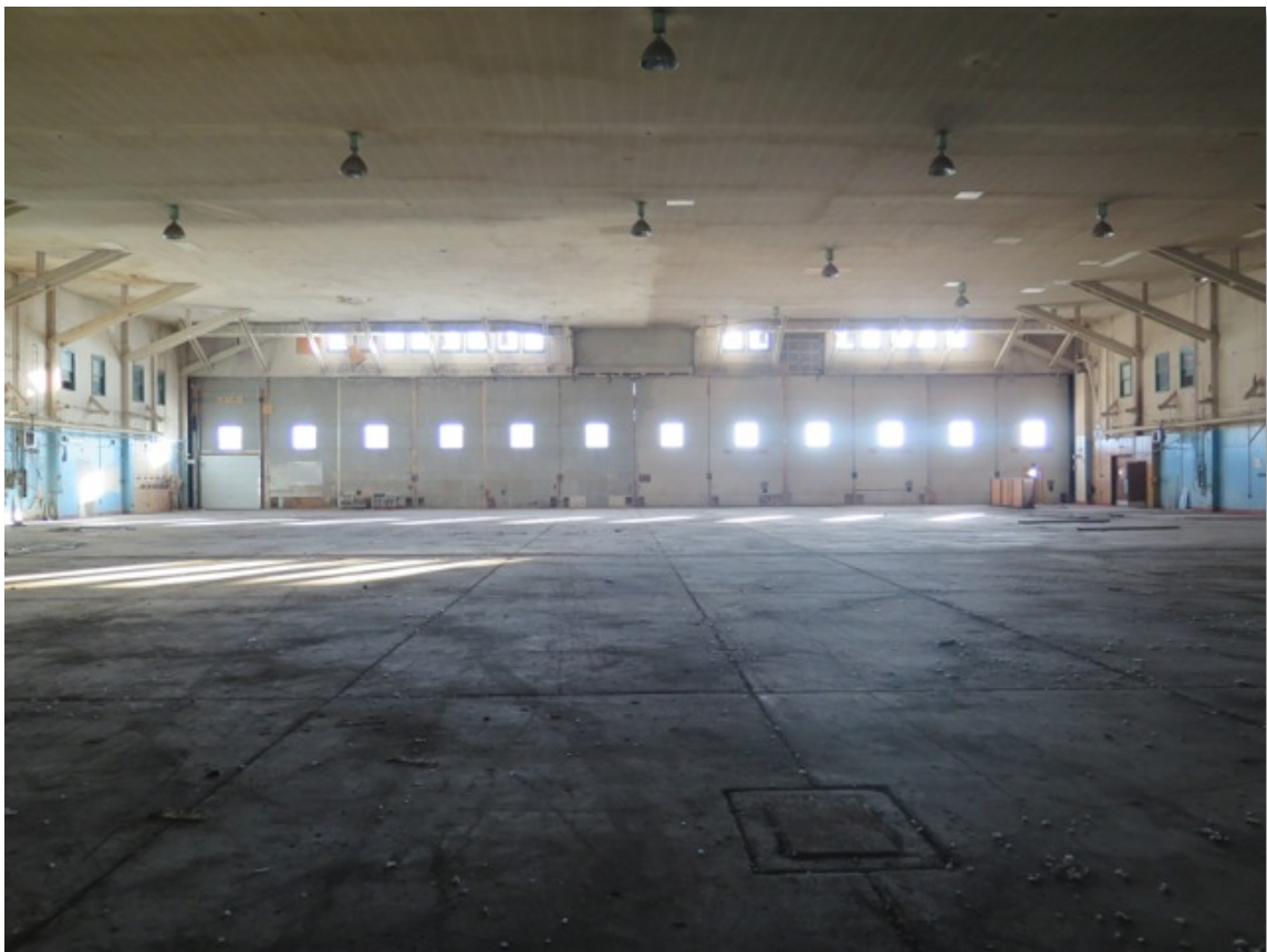
The interior of hangar 11 in 2017
