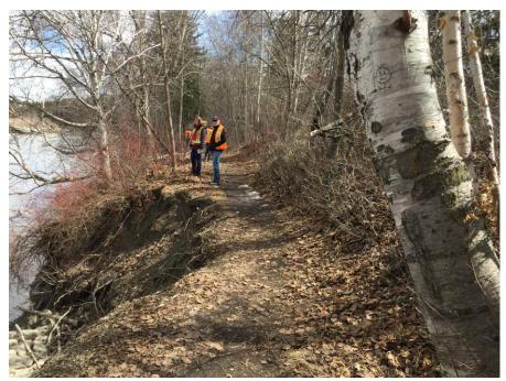
Plate 1.2. Slumping of the south bank of the NSR along Riverside Trail (Location 6) (22 April 2020).
