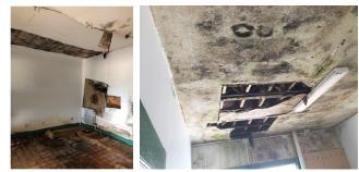
Photos 8 to 9: Ancillary Framing – Damaged Finishes due to water Infiltration
