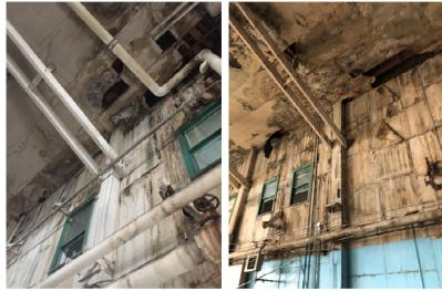
Photos 3 and 4: Hanger Walls – Signs of Deterioration
