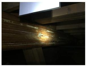
Photo 2: Chord - Potential glue deterioration
