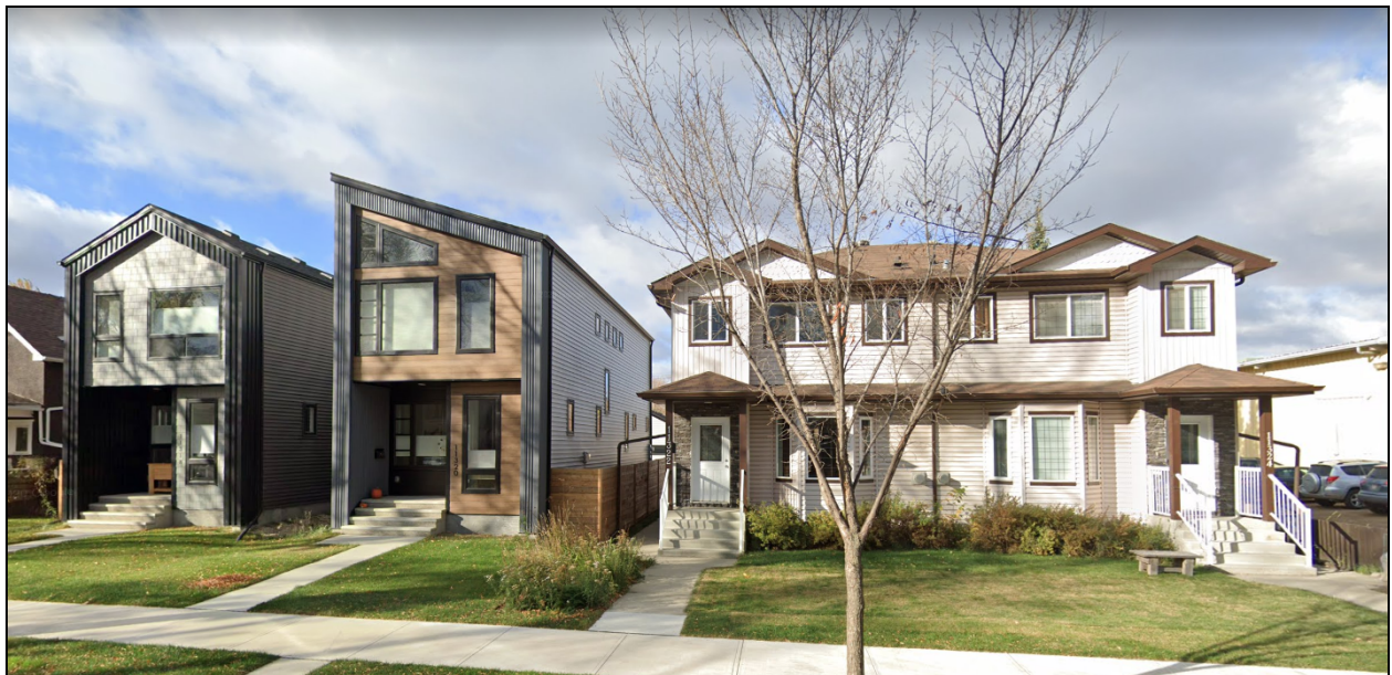
TYPICAL NEW RF3 + MNO DEVELOPMENT LOCATED ACROSS THE LANE TO THE EAST OF THE REZONING SITE
