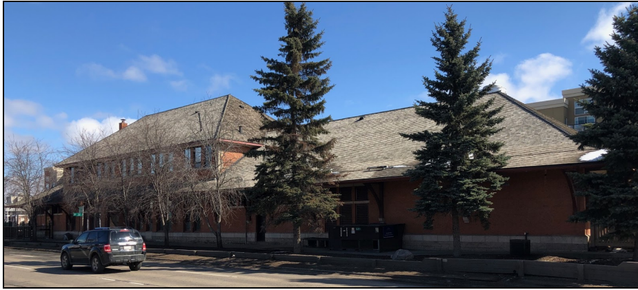
VIEW OF SITE LOOKING NORTHEAST SHOWING HISTORIC CANADIAN PACIFIC RAILWAY STATION
