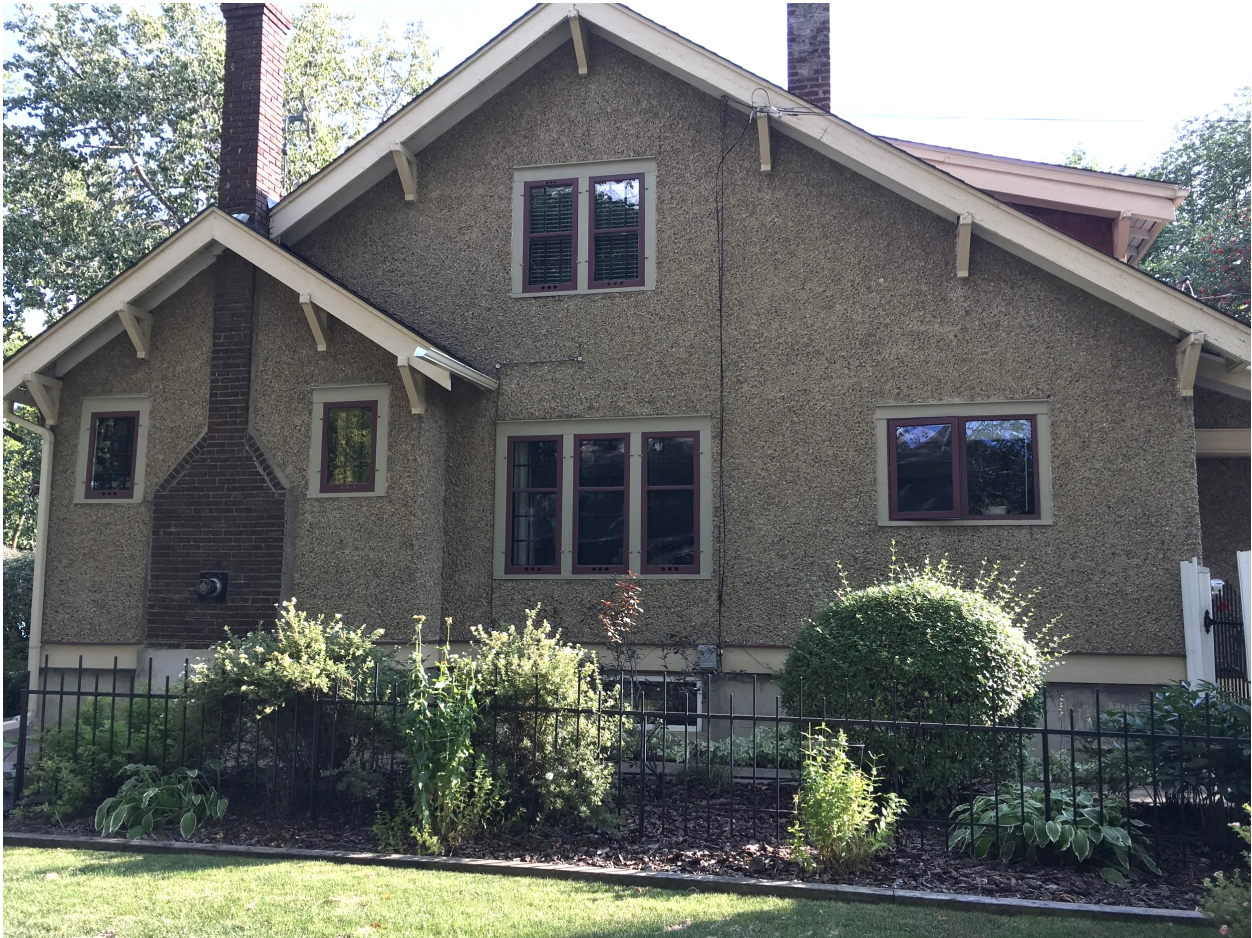
Photo #2 – Side (North) Elevation
