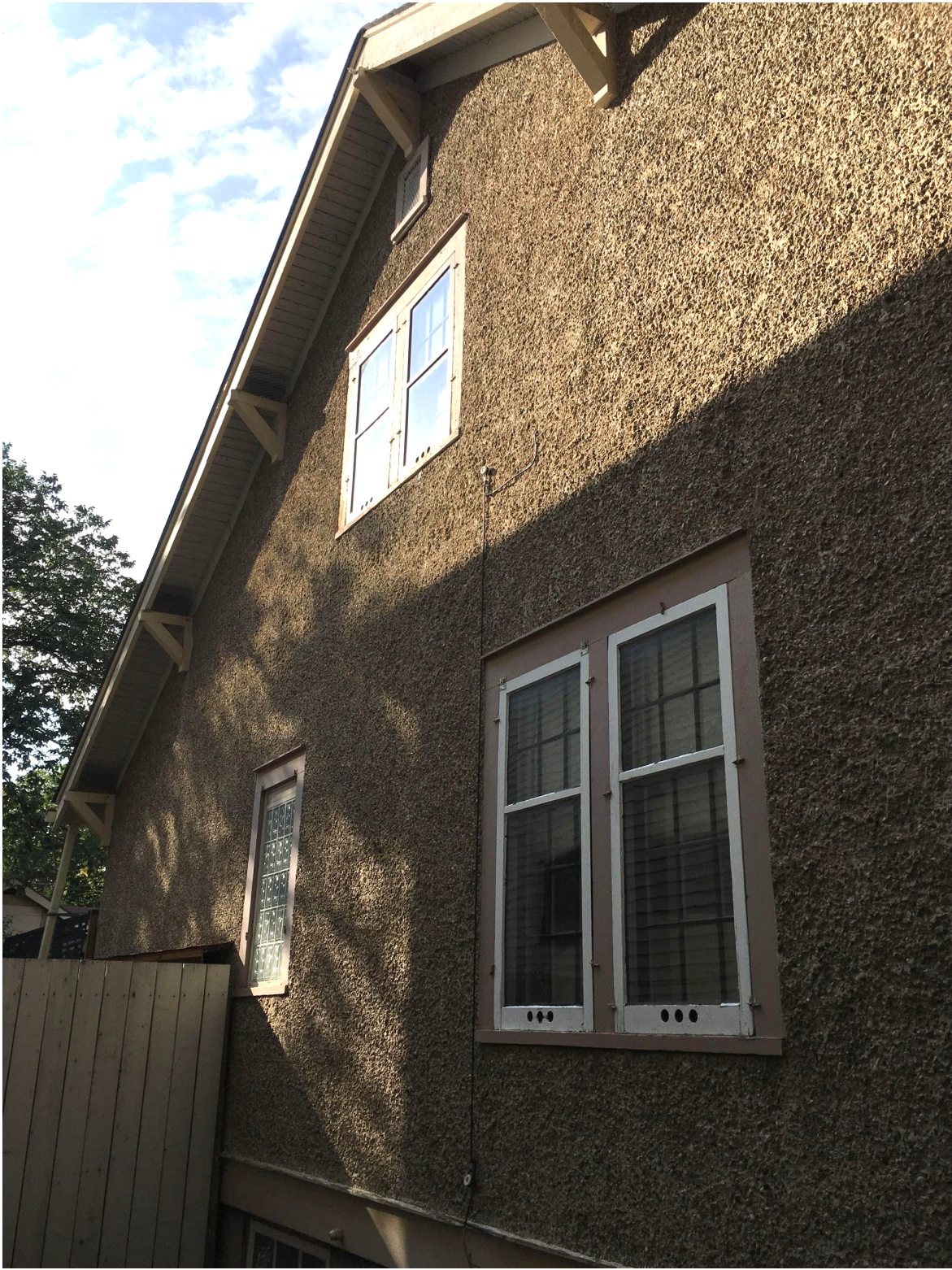
Photo #4 – Side (South) Elevation
