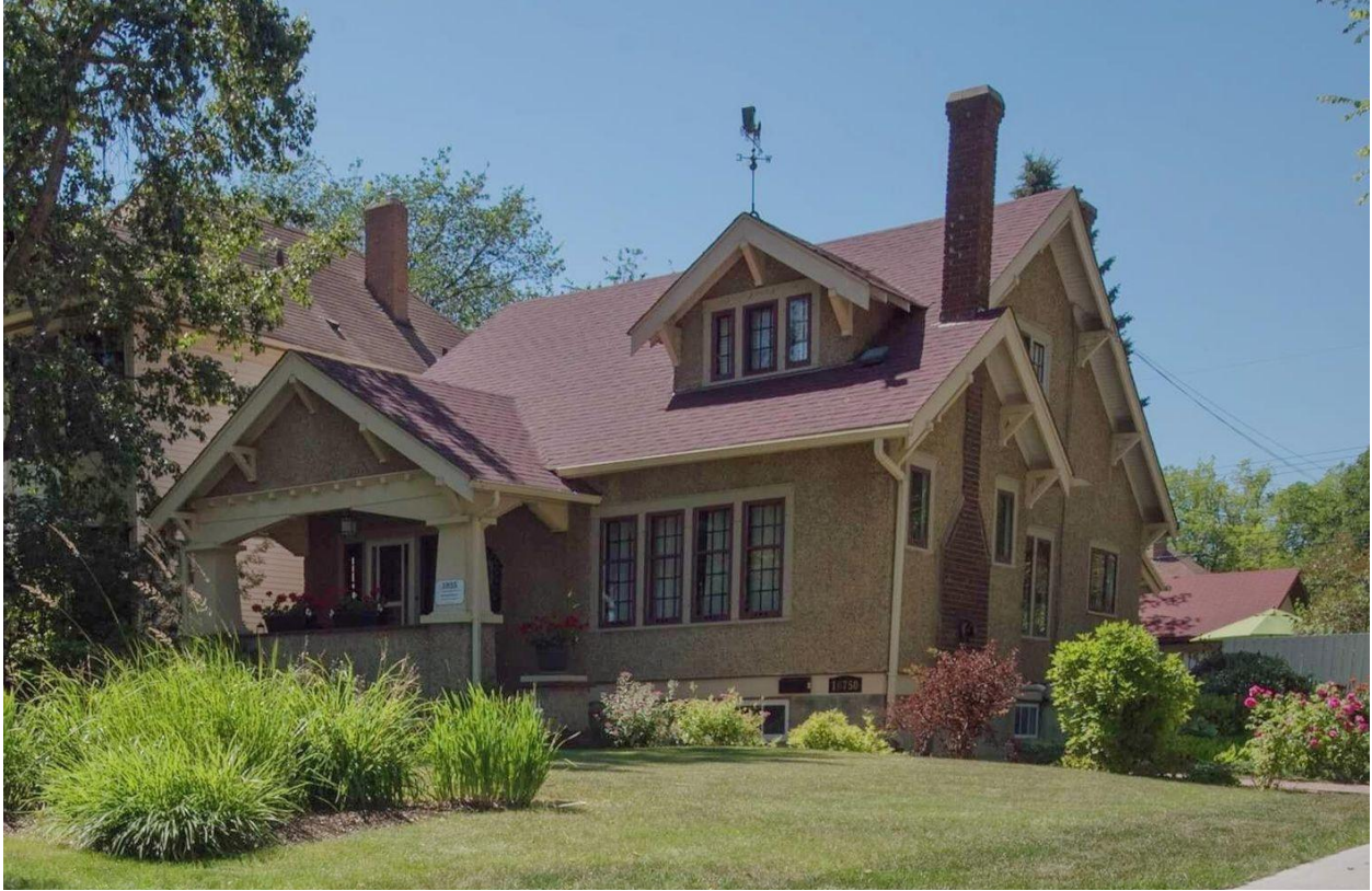
Photo #1 – Front (East) Elevation
