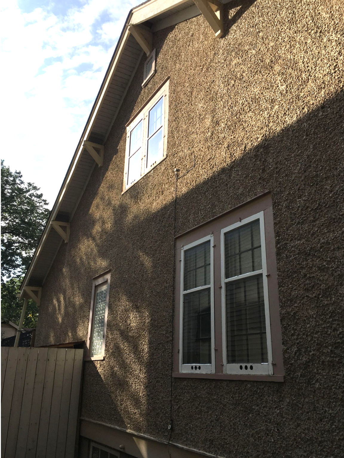
South Facade (side of house)
