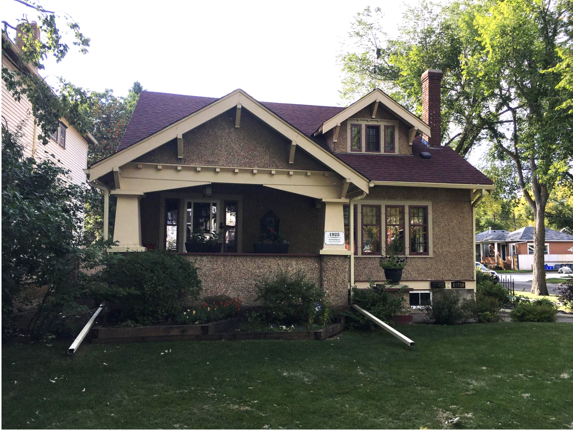
East Facade (front of house)
