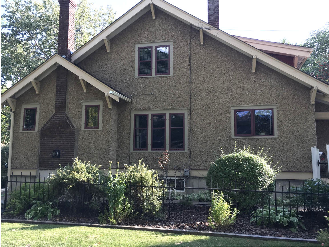
North Facade (side of house)
