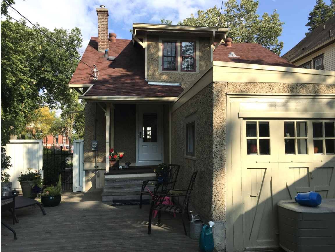
West Facade (back of house)
