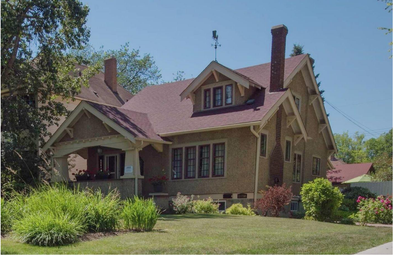
Photo #1 – Front (East) Elevation
