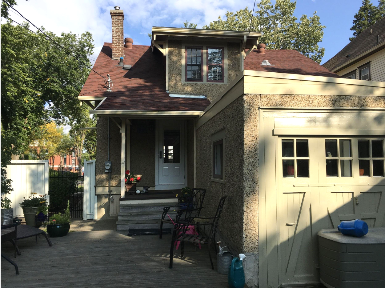
Photo #3 – Rear (West) Elevation
