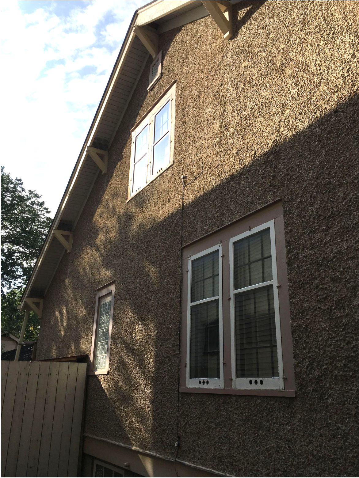
Photo #4 – Side (South) Elevation
