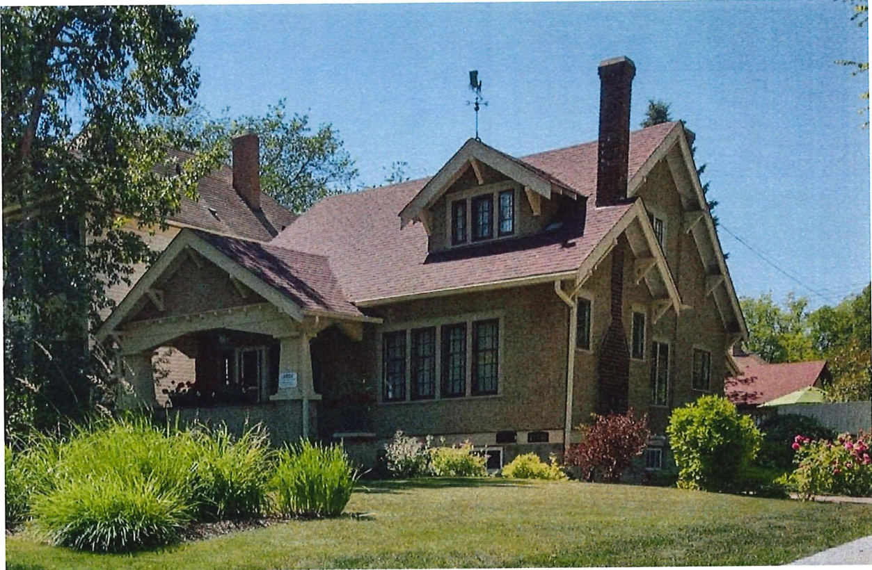
Photo #1 – Front (East) Elevation
