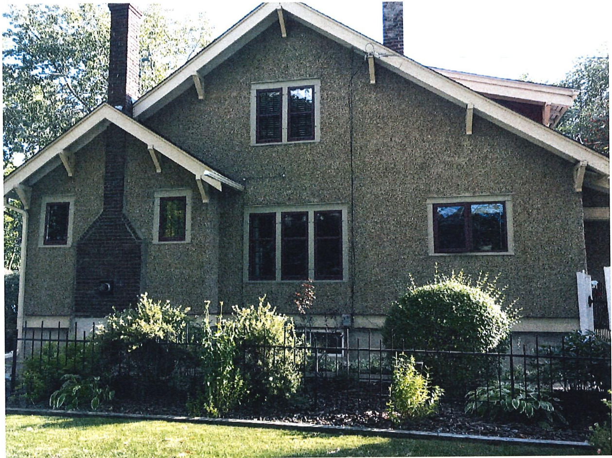
Photo #2 – Side (North) Elevation
