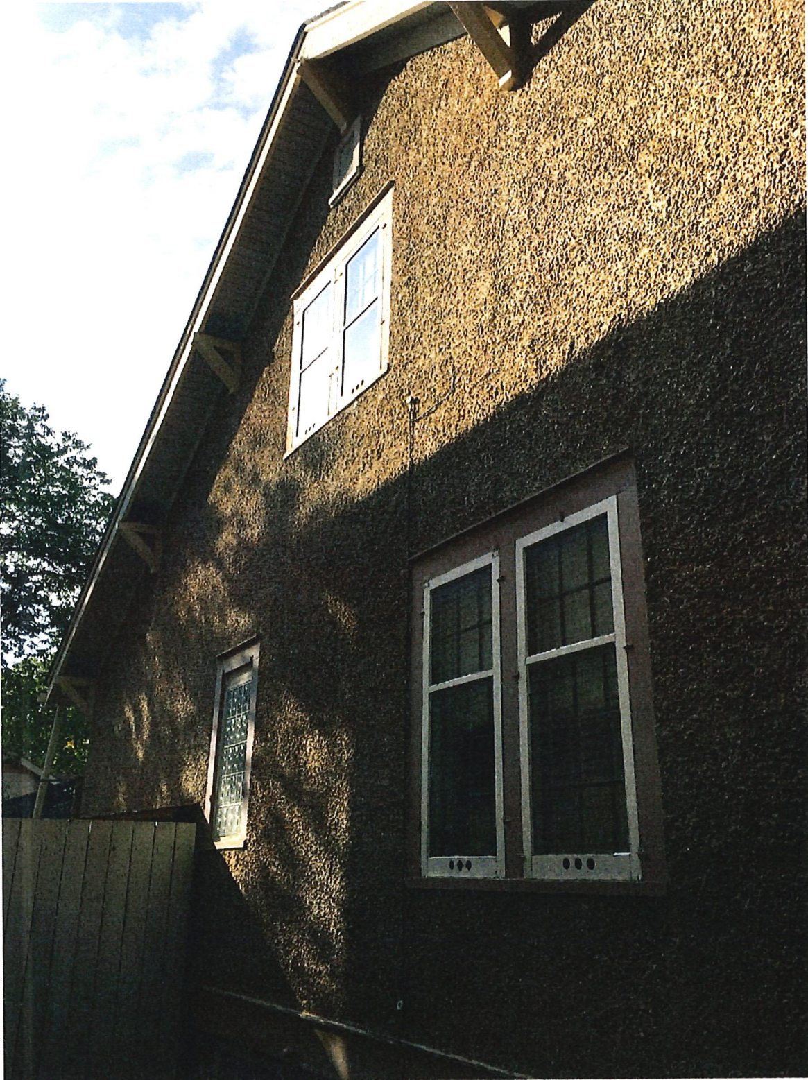
Photo #4 – Side (South) Elevation
