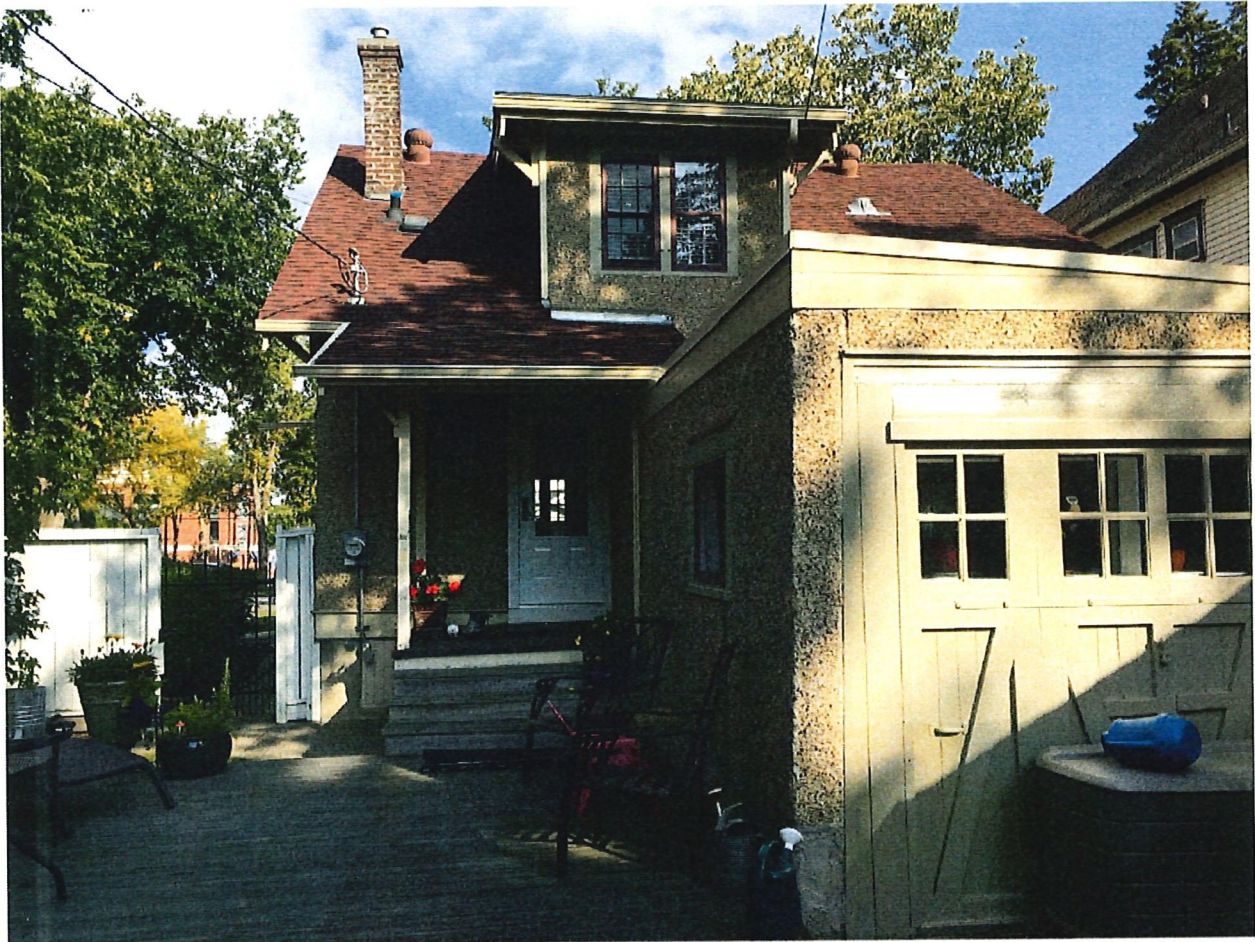
Photo #3 – Rear (West) Elevation
