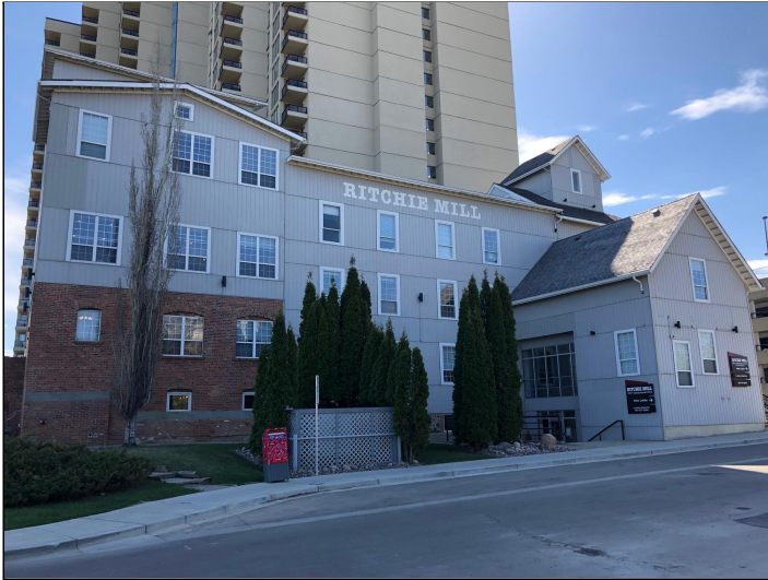
RITCHIE MILL - WEST FACADE
