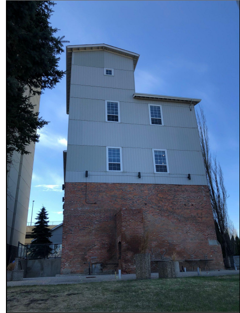
RITCHIE MILL - NORTH FACADE
