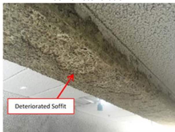
Figure 2.0-2 Soffit Deterioration
