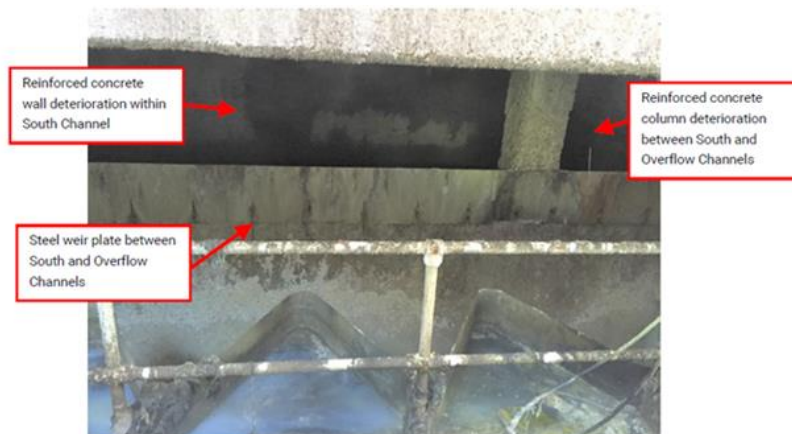
Figure 2.0-1 Concrete Deterioration
