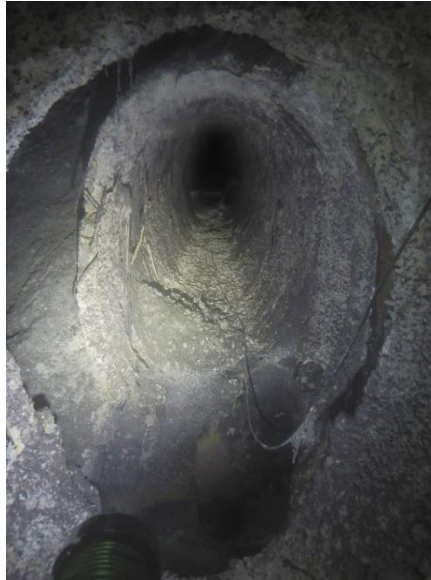
Figure 2.1-2 Large Void Upstream of Reach 49
