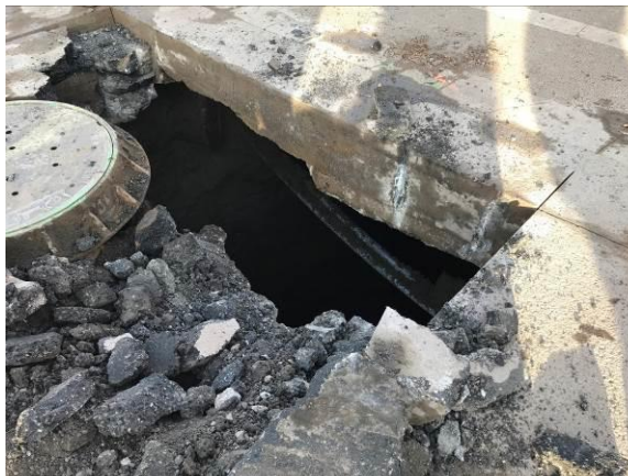
Figure 2.0-2 Severe Deterioration of 61 Avenue Trunk
