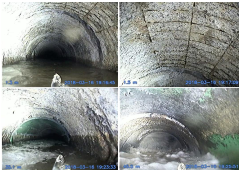
Figure 2.0-4 Deterioration of Small Trunks
