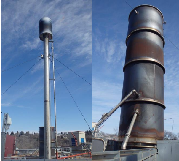
Figure 2.0-2 Candle Stick Flare (left) and Enclosed Burner Flare (right)
