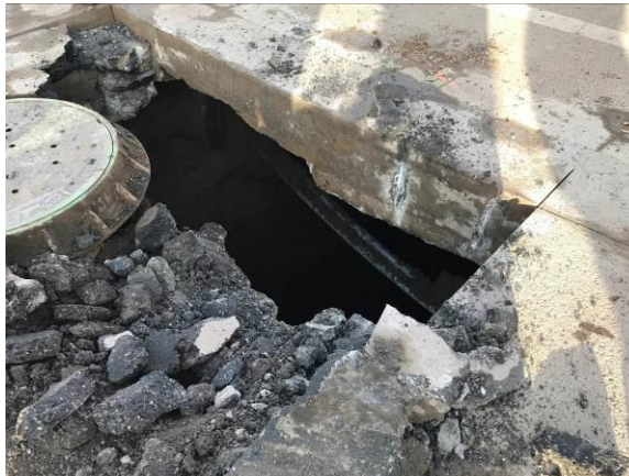
Figure 2.0-2 Severe Deterioration of 61 Avenue Trunk
