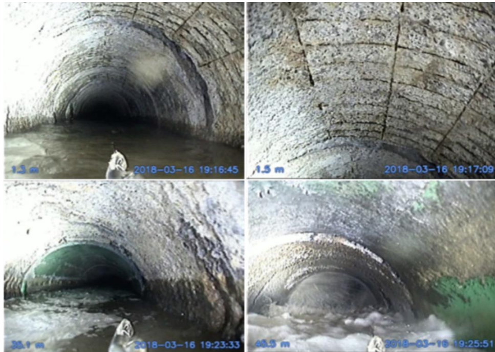
Figure 2.0-4 Deterioration of Small Trunks
