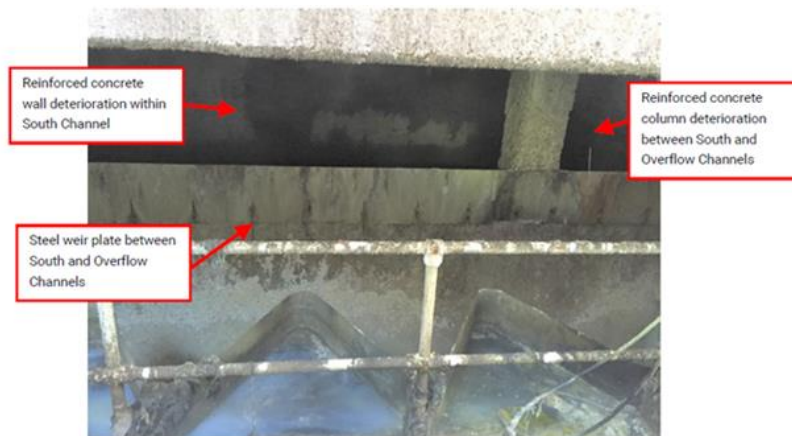
Figure 2.0-1 Concrete Deterioration
