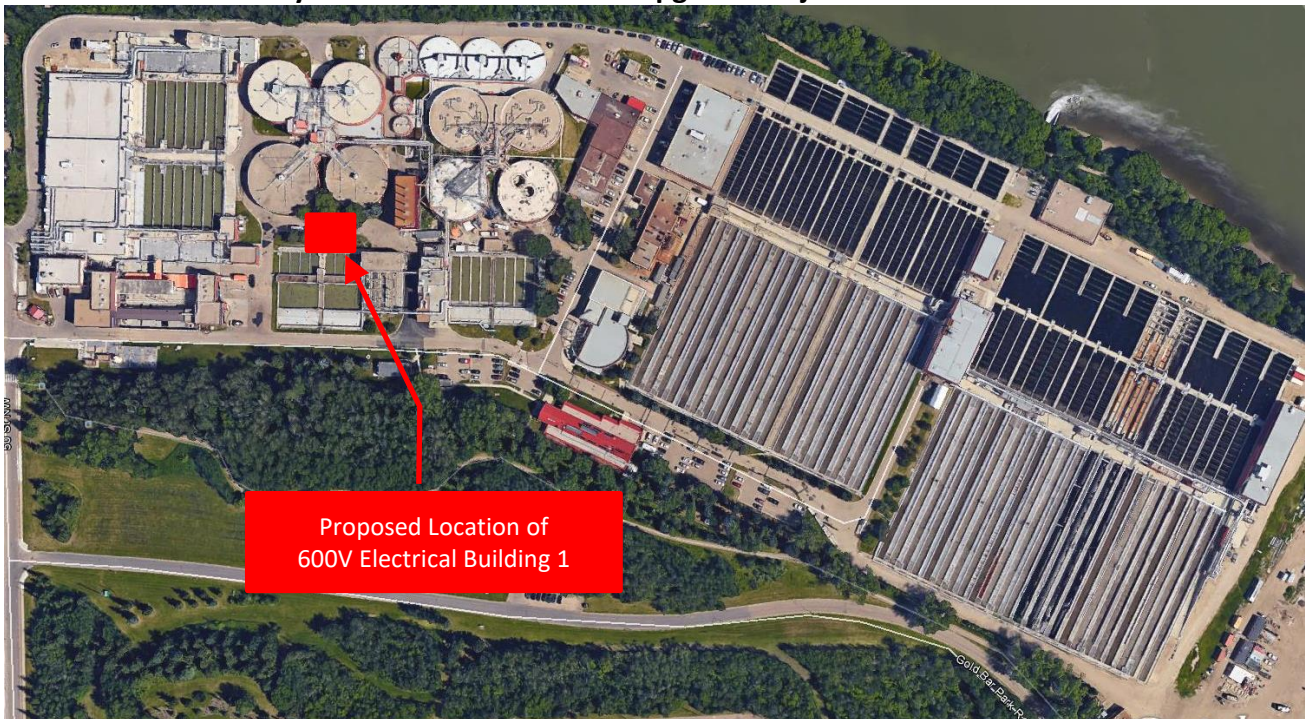
Figure 2.0-1 Auxiliary Control Room Electrical Upgrade Project Site Location Overview
