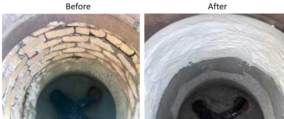
Figure 2.0-1 Typical Manhole Before and After Relining
