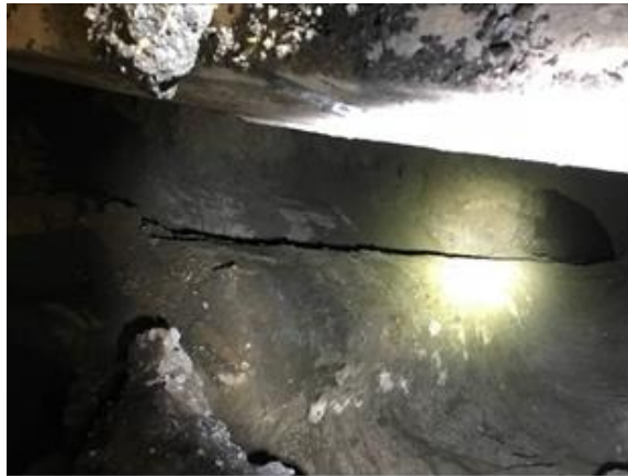
Figure 2.0-2 Severe Deterioration of 61 Avenue Trunk
