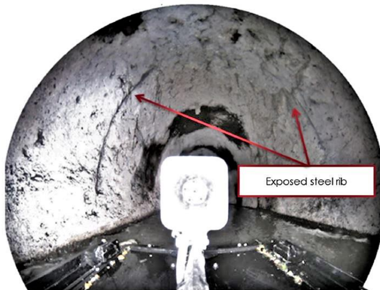
Figure 2.2-1 Photo Condition of 99 Avenue Trunk
