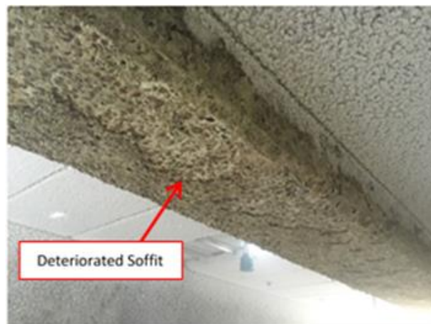
Figure 2.0-2 Soffit Deterioration
