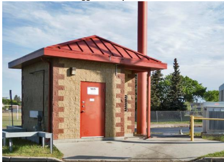
Figure 2.0-3 Duggan Pump Station
