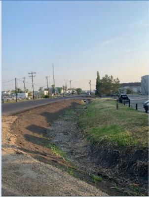
Majority of ditches were overgrown resulting in blocked flow paths. Vegetation was cleared and culverts repaired to increase flow capacities. New grass seed is being applied and will be maintained annually to maintain drainage functionality
