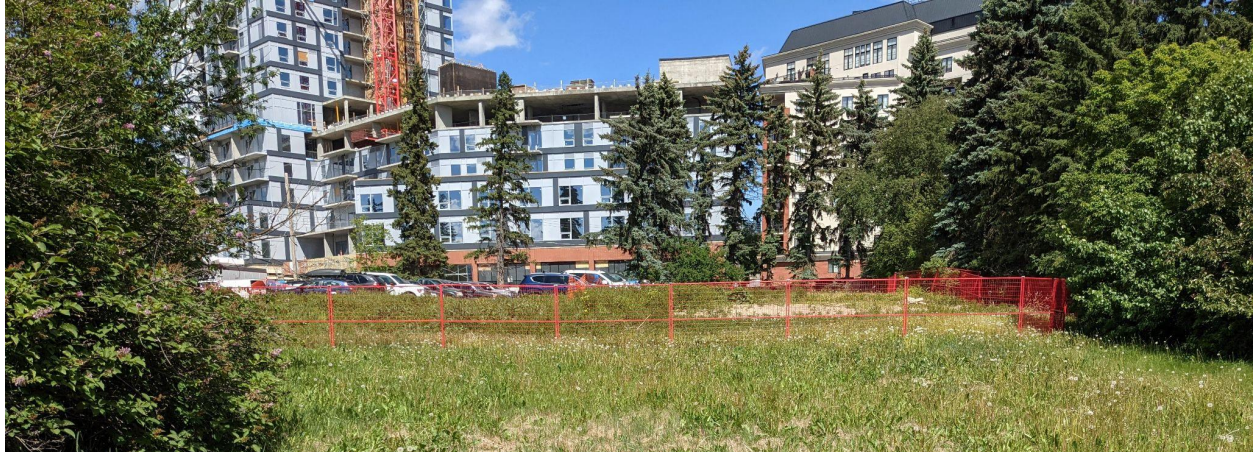
PHOTO OF SITE (WITHIN RED FENCE) FROM WEST (GROAT RAVINE SIDE)
