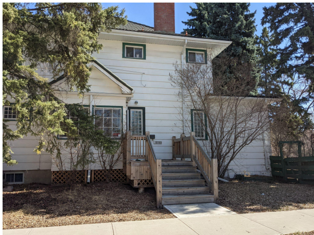
VIEW OF SITE FROM WEST
