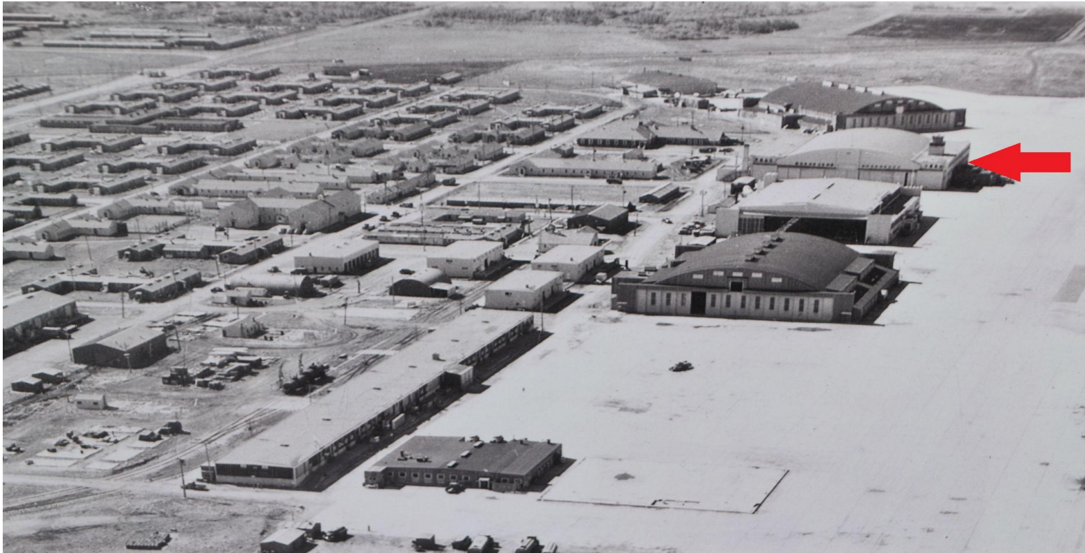
Hangar 11, with red arrow, 1945
