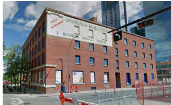
LOOKING NORTHEAST FROM 103 AVENUE NW
