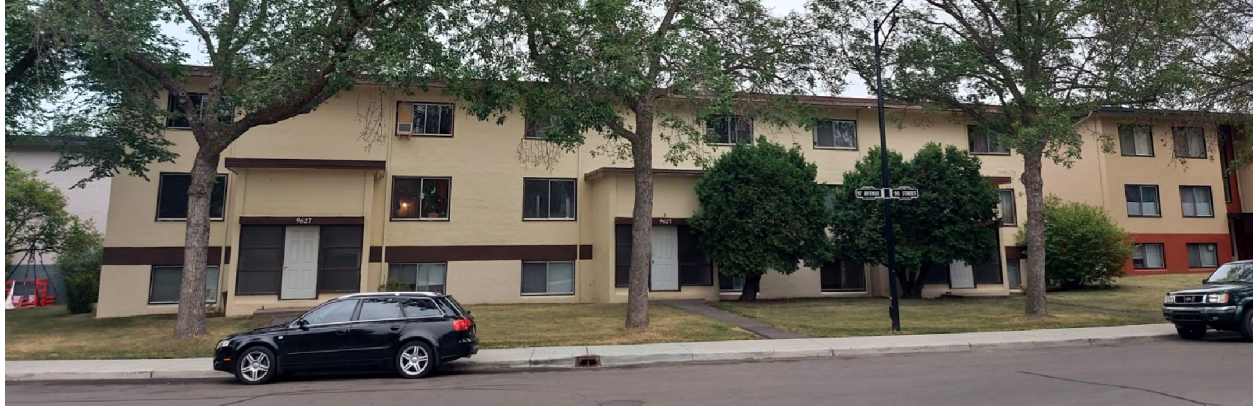
VIEW OF THE SITE AND EXISTING LOW RISE APARTMENTS LOOKING EAST ACROSS 90 STREET
