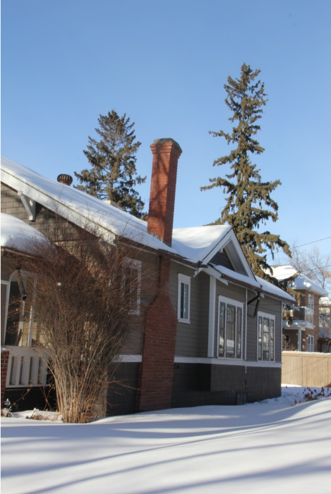
Photo #2 – East elevation, viewed from 109A Avenue NW (2018)
