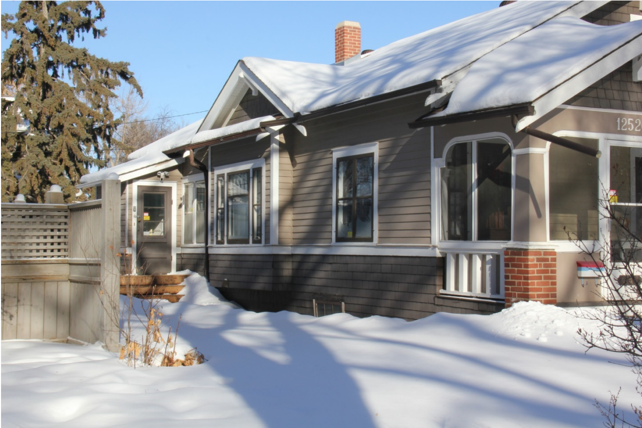
Photo #4 –West elevation, viewed from 109A Avenue NW (2018)
