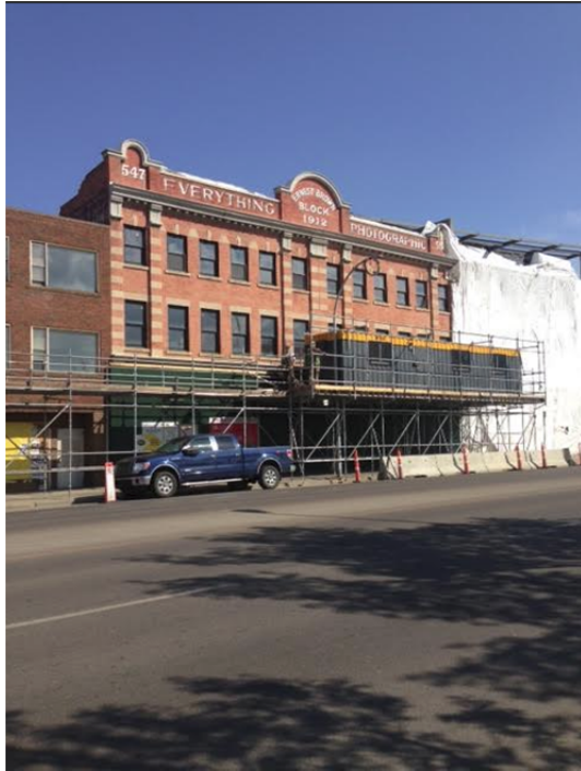
VIEW FROM JASPER AVENUE NW, FACING NORTHEAST
