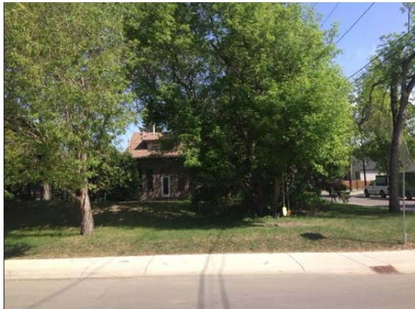
VIEW FROM 101 AVENUE NW, FACING NORTH
