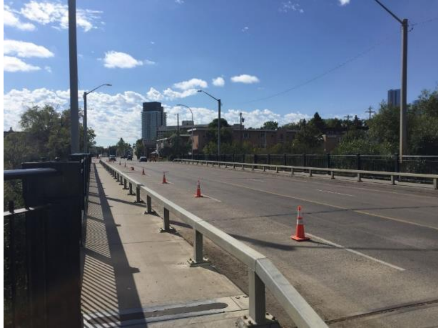
Plate 1.1. View to southwest of Latta Bridge on Jasper Avenue (11 September 2020).
