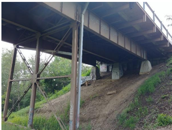
Plate 1.3. View to southeast under Latta Bridge (02 August 2019).
