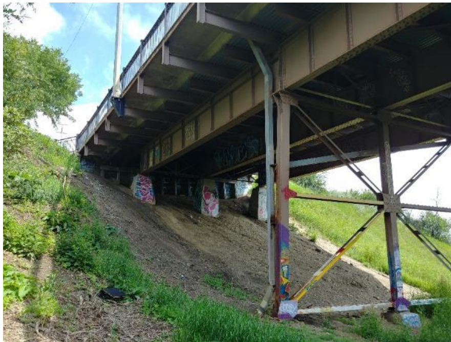
Plate 1.2. View to northeast under Latta Bridge (02 August 2019).
