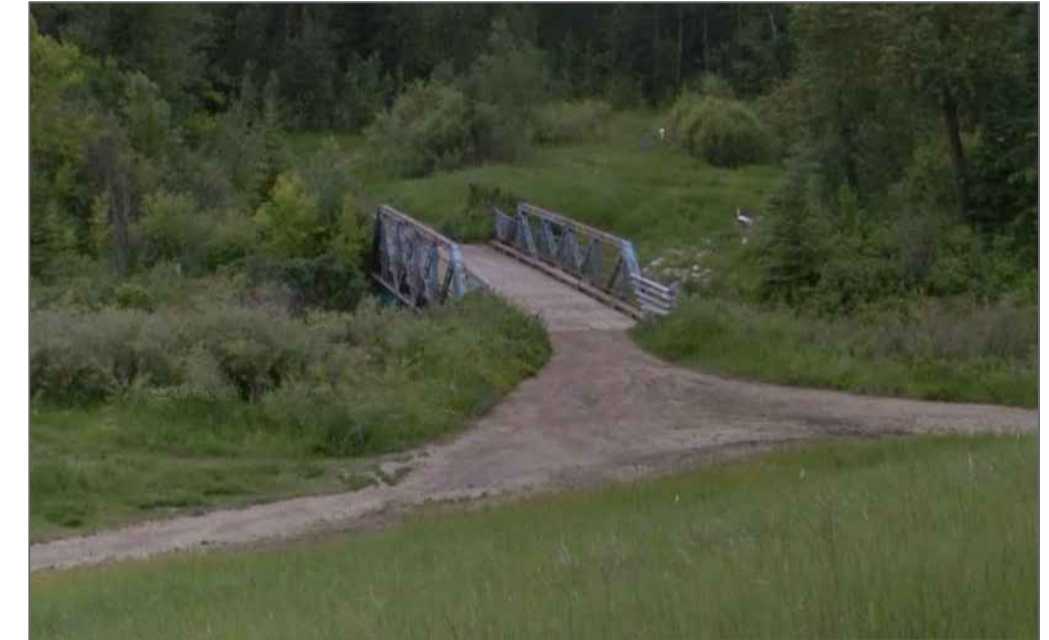
EXISTING BRIDGE PHOTO
