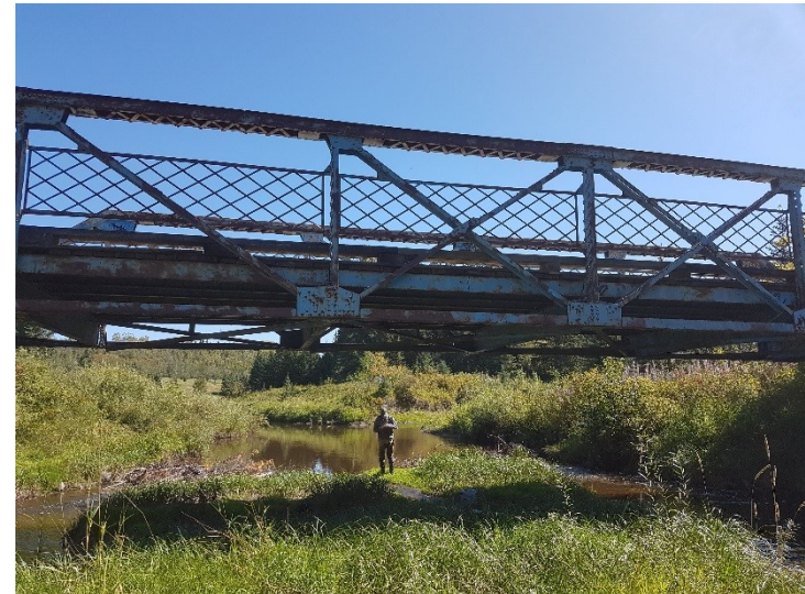
Plate 4: Looking upstream at the bridge structure.
