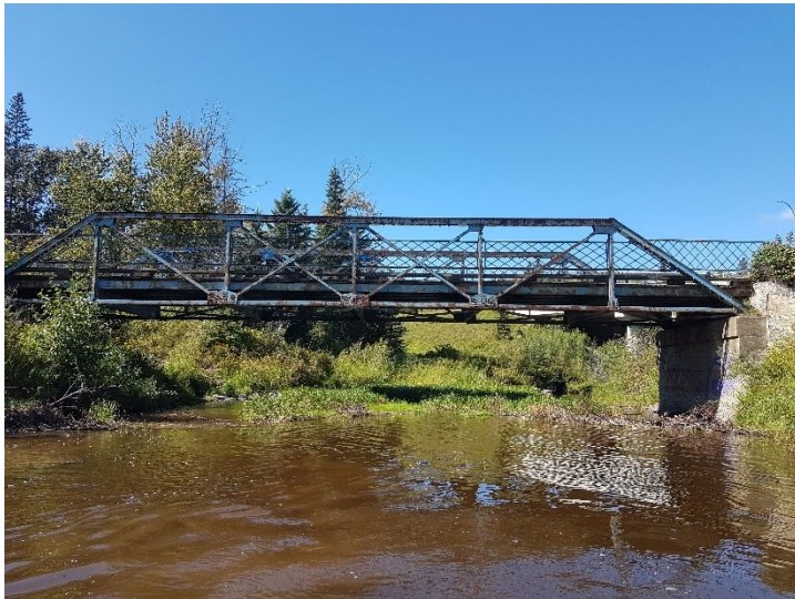
Plate 3: Looking downstream at the bridge structure.
