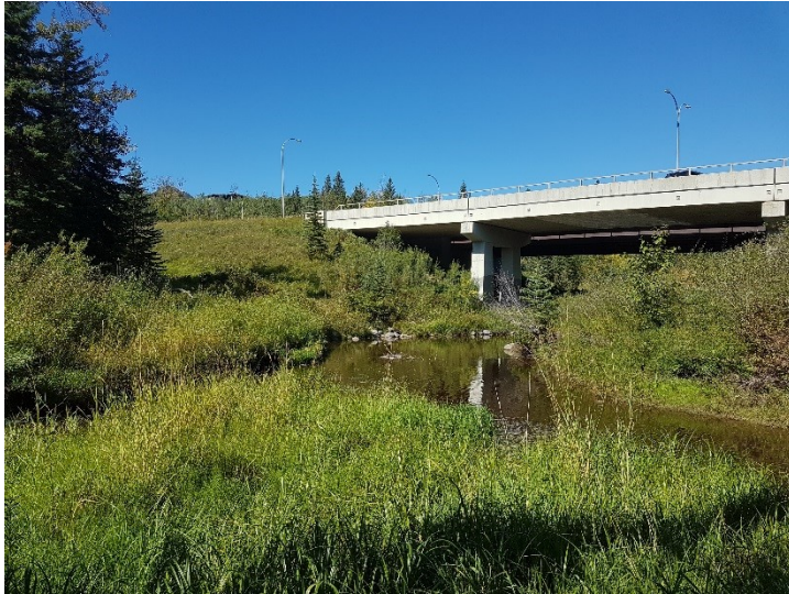
Plate 5: Looking downstream from below the bridge structure.
