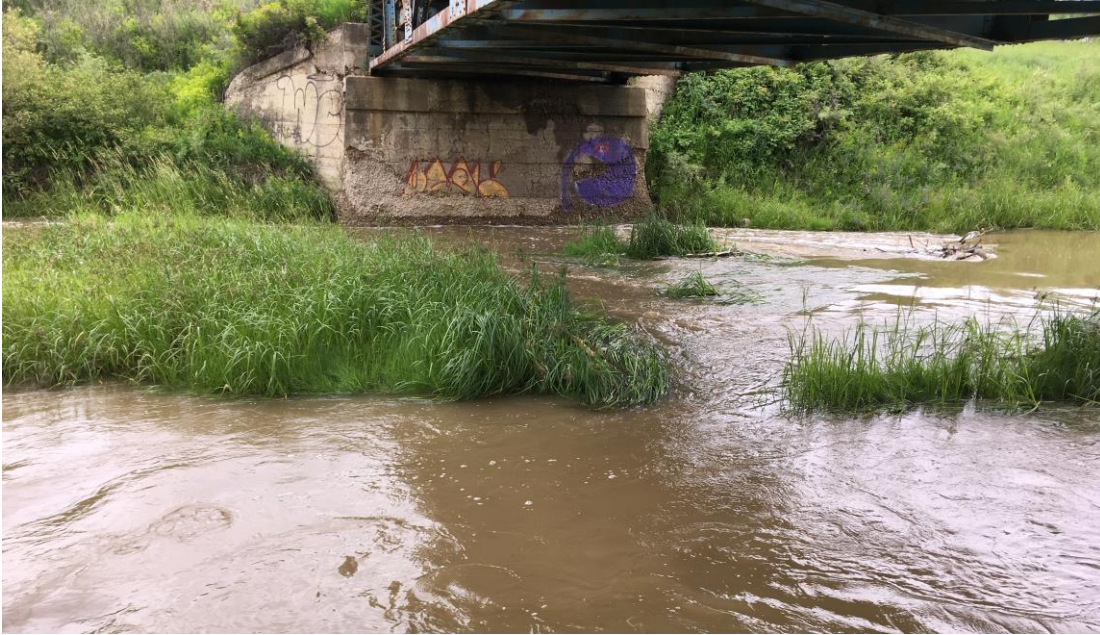
Photo 3 – View of Existing North Abutment (Looking North)
