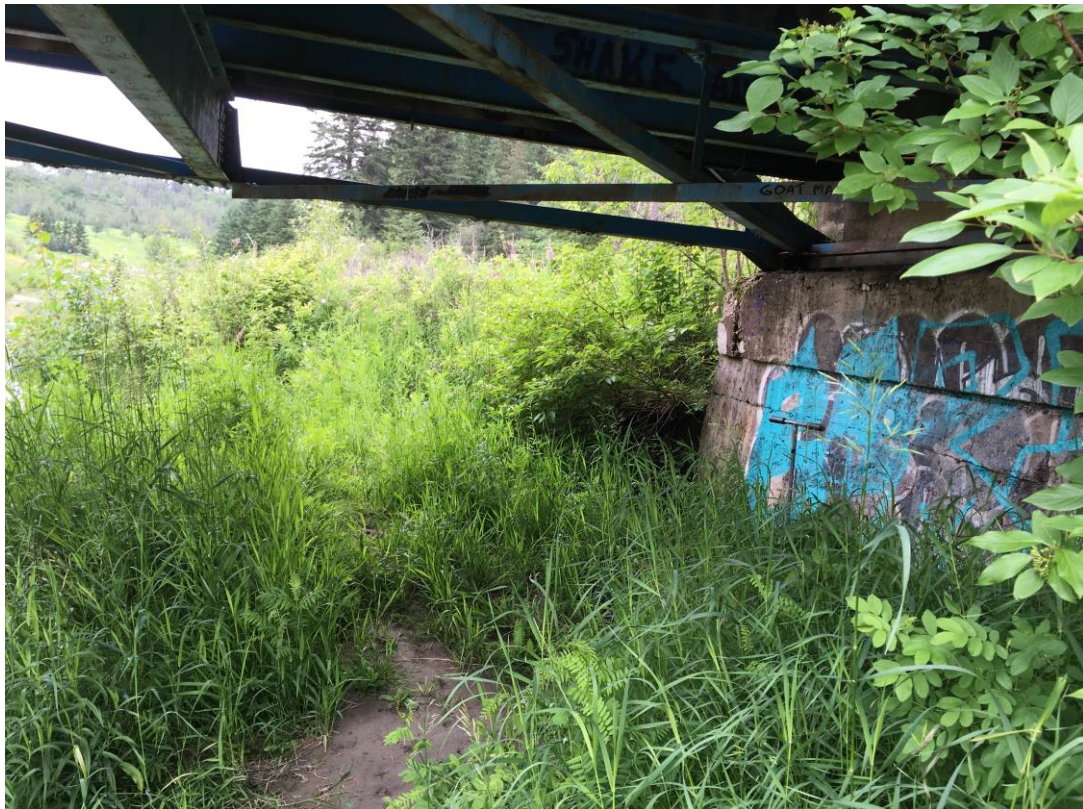
Photo 4 – View of Existing South Abutment (Looking from East)
