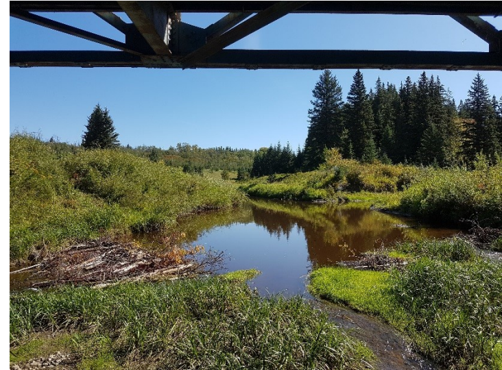
Plate 6: Looking upstream from below the bridge structure.
