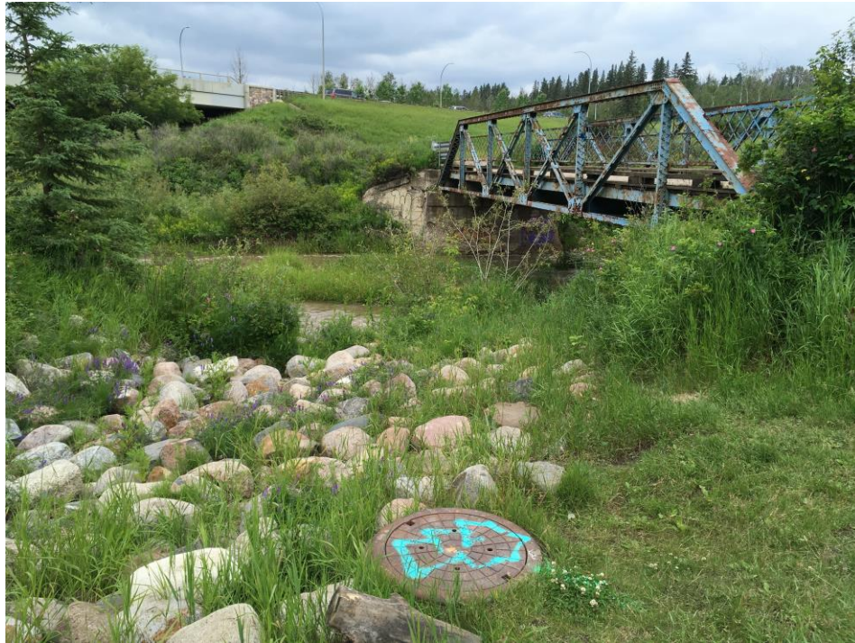
Photo 1 – View of Smith Crossing Bridge (Looking North).
