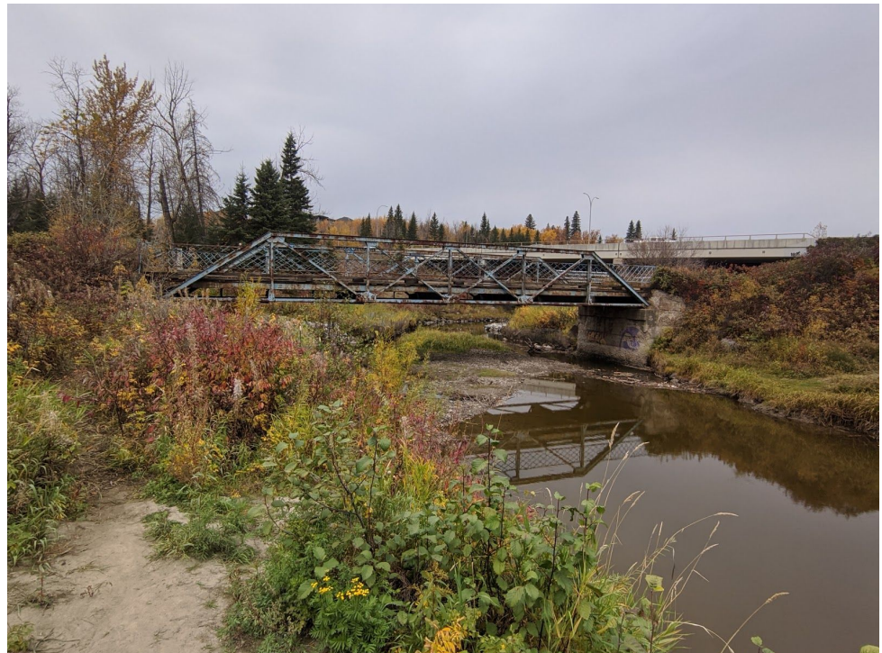
Existing Smith Crossing Pedestrian Bridge - looking west in fall 2020
