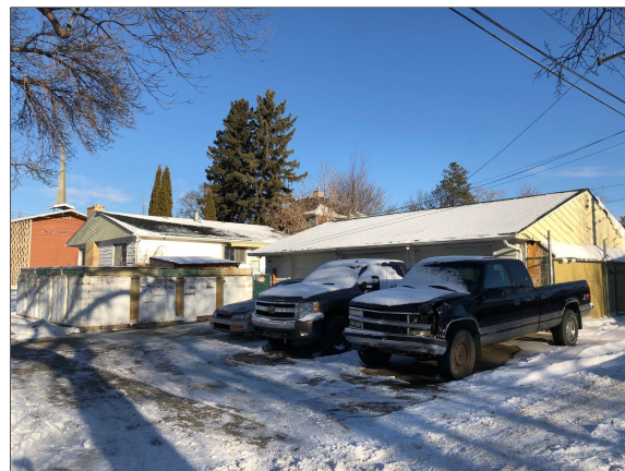
VIEW OF SITE LOOKING NE FROM 86 STREET NW
