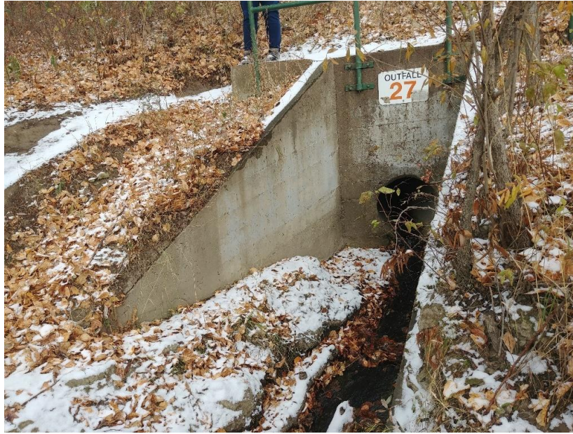
Plate 2.3. Hawrelak Park Stormwater Outfall 27 (erosion and concrete work to increase bank stability; pipe condition does not warrant replacement) on east bank of NSR downstream of the Pumphouse (20 October 2020).
