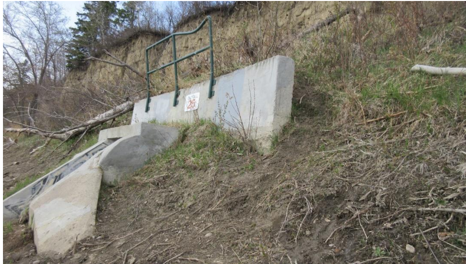
Plate 2.5. Hawrelak Park Stormwater Outfall 25 (replace pipe; concrete outfall structure in good condition, no works required) on the East Bank of the North Saskatchewan River (12 May 2021)
