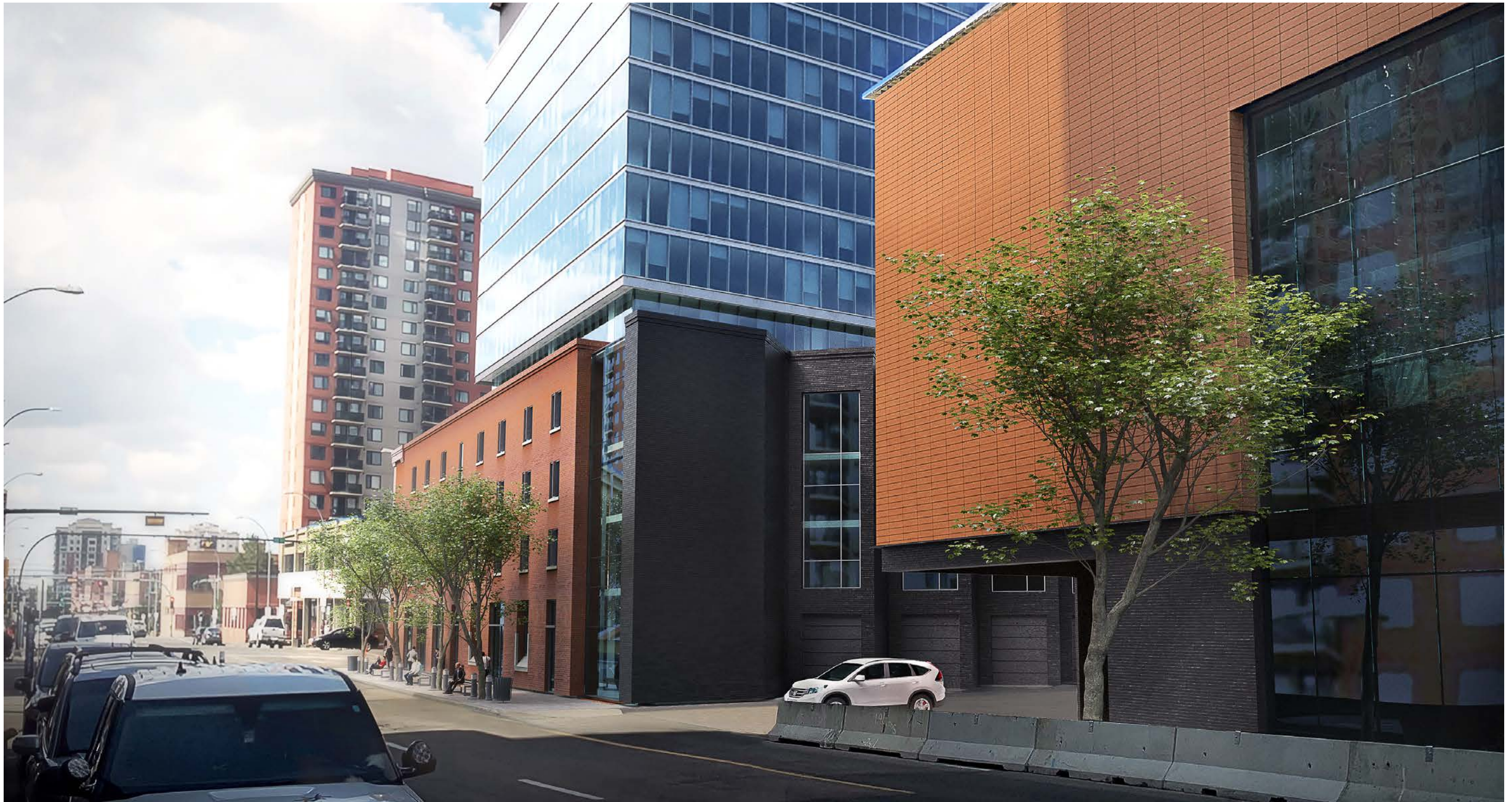
View looking West along 103 Ave NW
