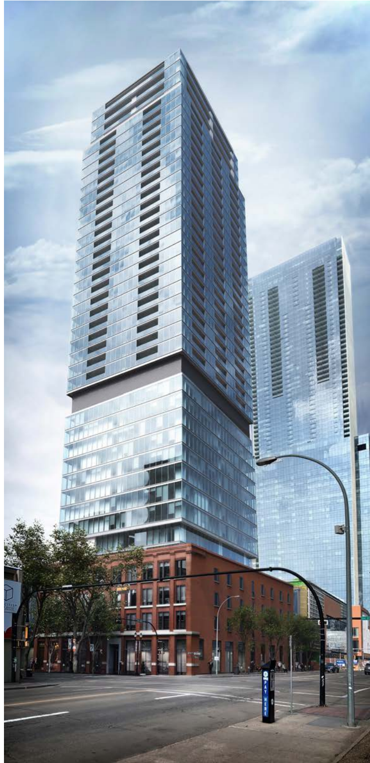
View looking East along 103 Ave NW
