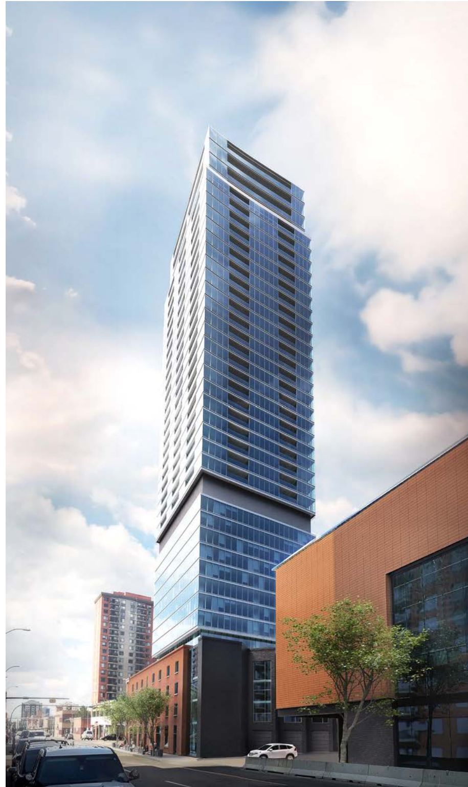
View looking West along 103 Ave NW
