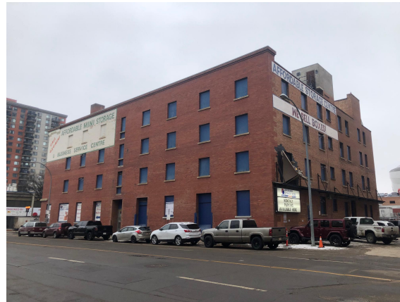
View of the site looking northwest from 103 Avenue NW
