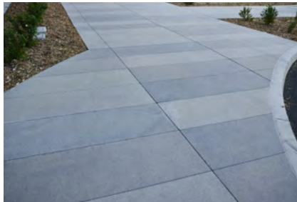
decorative concrete finish
