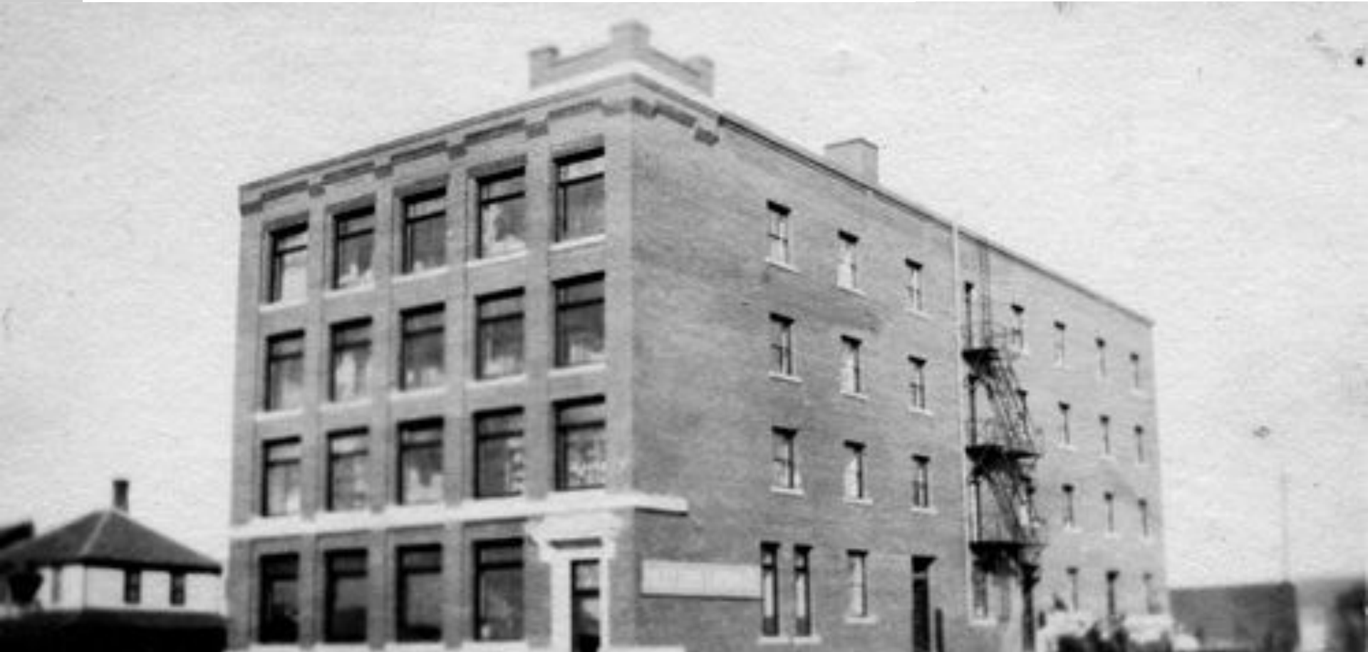
HORNE & PITFIELD BUILDING. CITY OF EDMONTON ARCHIVES EB-38-3
