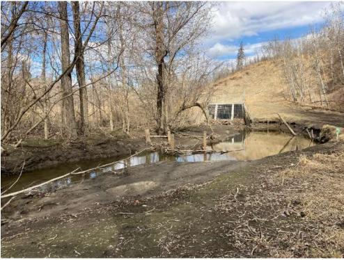
Figure 2-1: Looking at EPCOR Inlet Structure (Note; Debris catcher in channel and debris blockage at inlet screen (April 19, 2021 site visit photo)
