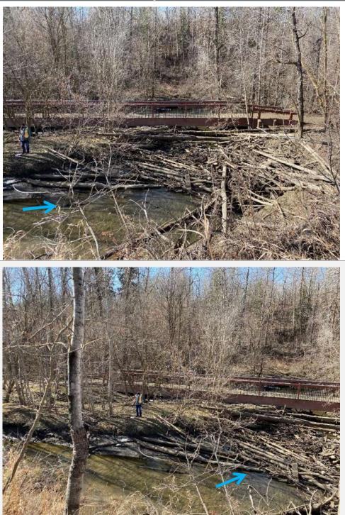
Photo 1 Looking downstream (southwest) at the west section of the bridge B278. Note the accumulated debris upstream of the bridge. Also note that Mill Creek main channel is only under the west bridge span.
