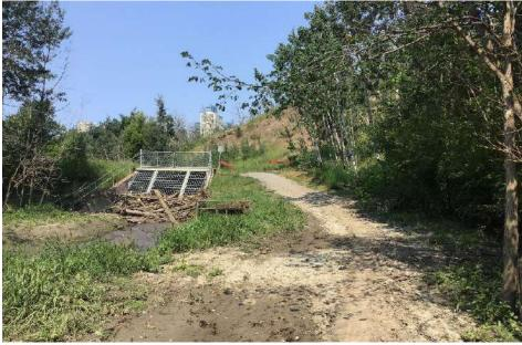
Plate C11: July 27, 2021. Facing downstream (northwest) from the pedestrian trail approximately 55 m north of B278, showing woody denris jam at the EPCOR inlet structure.
