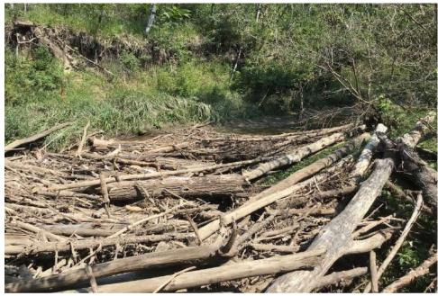
Plate C1: July 27, 2021. Facng upstream (east), from 2 m upstream of B278, showing steeply eroded and slumping right (east) bank. Note woody denris jam at B278 bridge opening.
