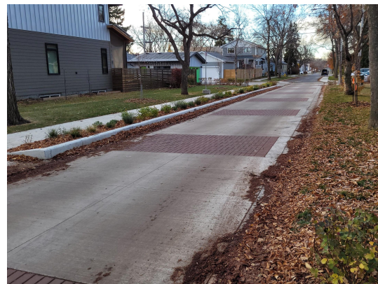
98 St between 84 and 85 Avenue
