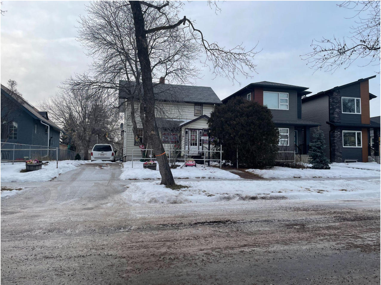
View of the site looking northwest from 108 Street NW
