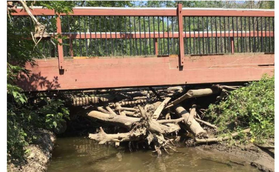
Plate C12: July 27, 2021. Facing upstream (northeast) from downstream of B278, showing pool habitat with fine textured substrate material at the crossing. Note woody debris jam and rock filled gabion basket on the right bank, at the crossing.
