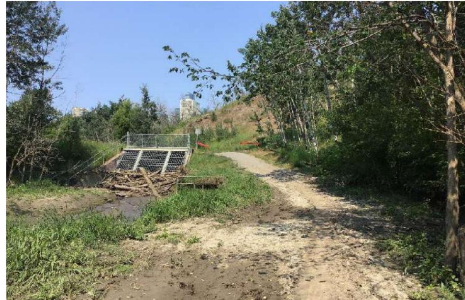
Plate C11: July 27, 2021. Facing downstream (northwest) from the pedestrian trail approximately 55 m north of B278, showing woody debris jam at the EPCOR inlet structure.
