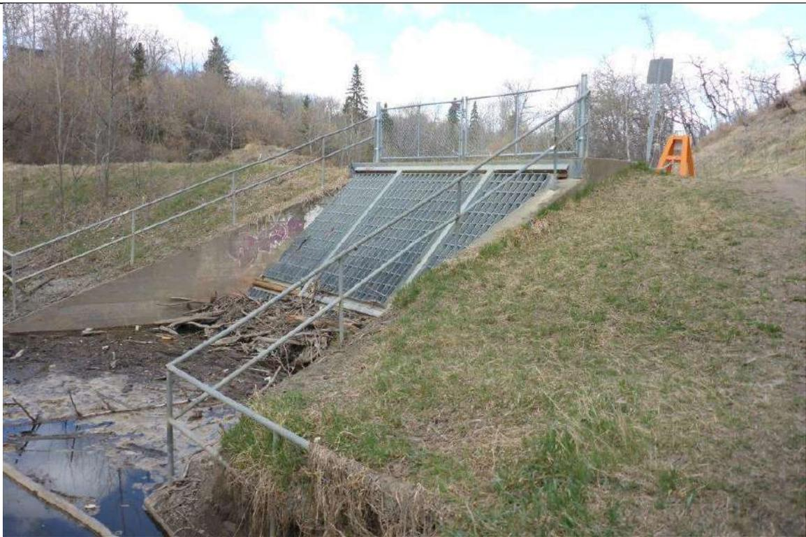
Photograph 2: Inlet structure connecting Mill Creek Ravine to the North Saskatchewan River.
