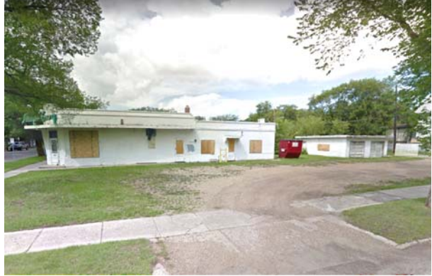
VIEW OF SITE LOOKING WEST FROM 116 STREET NW
