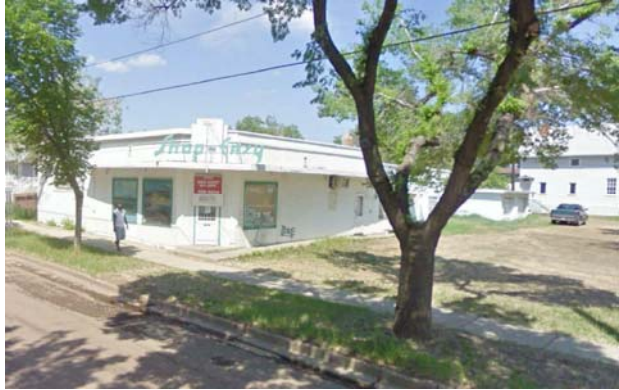
VIEW OF SITE LOOKING NORTH FROM 129 AVENUE NW
