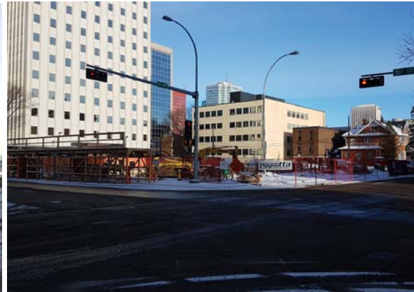
VIEW OF SITE FACING NORTHEAST
