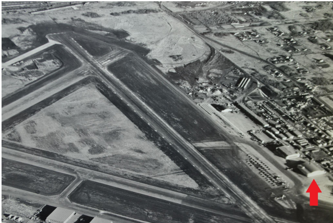
Hangar 11, shown with red arrow, 1943, looking northeast.
