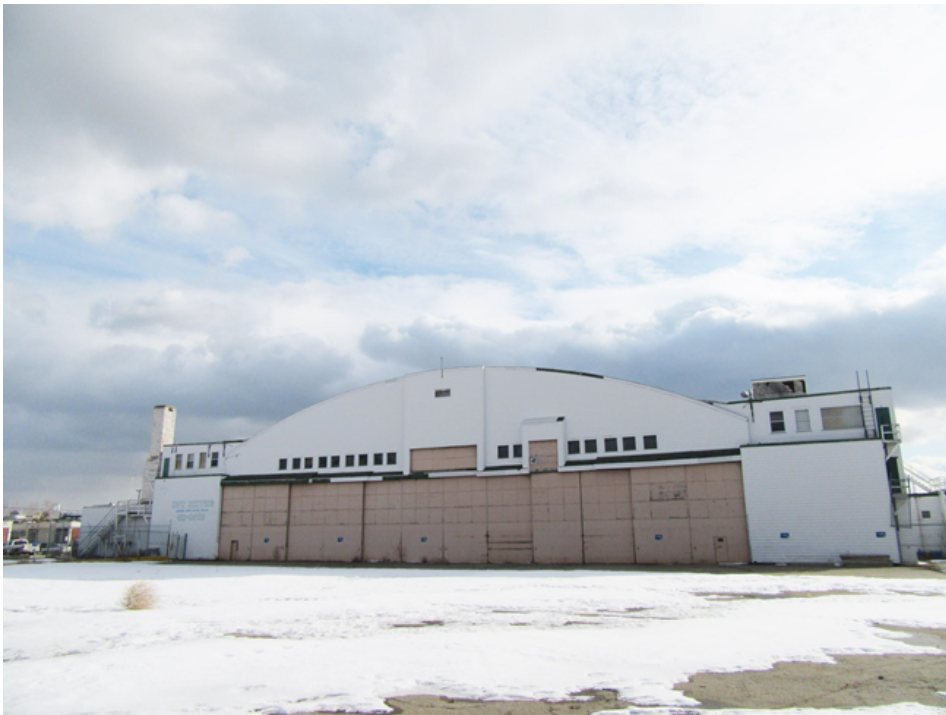
Hangar 11, north elevation, looking southeast from Blatchford site.
