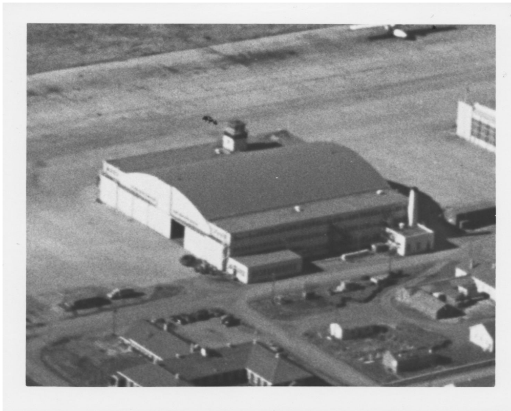
Hangar 11, 1943, looking northwest.
