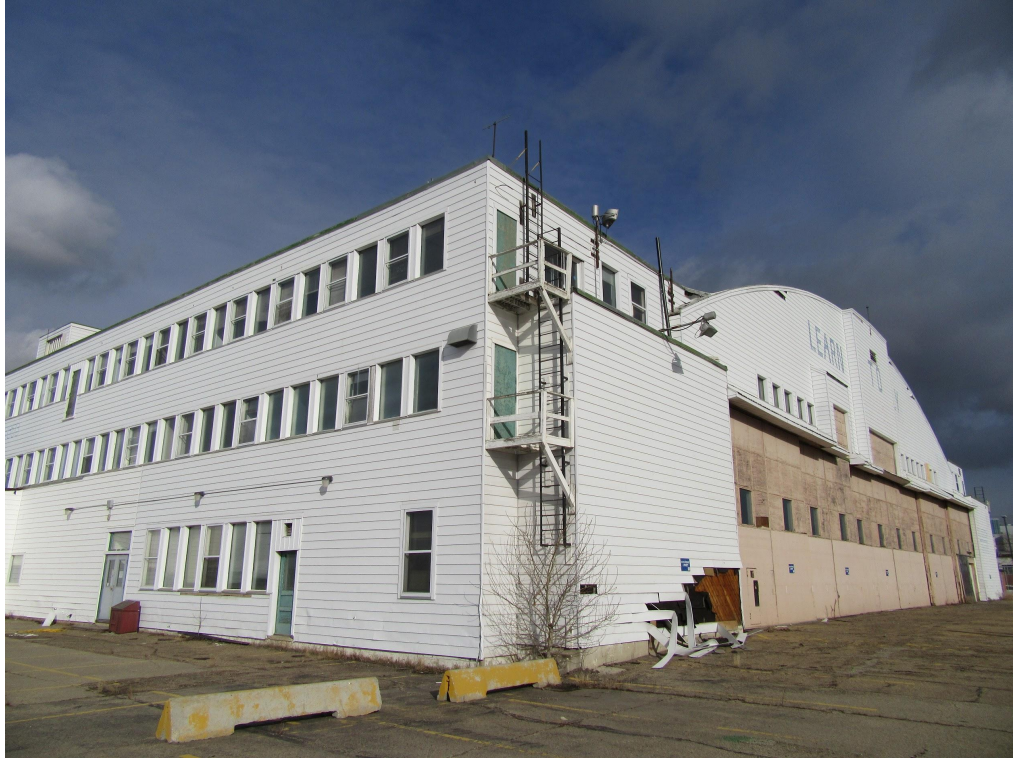
Hangar 11, south and west elevations, looking northeast from Blatchford site.
