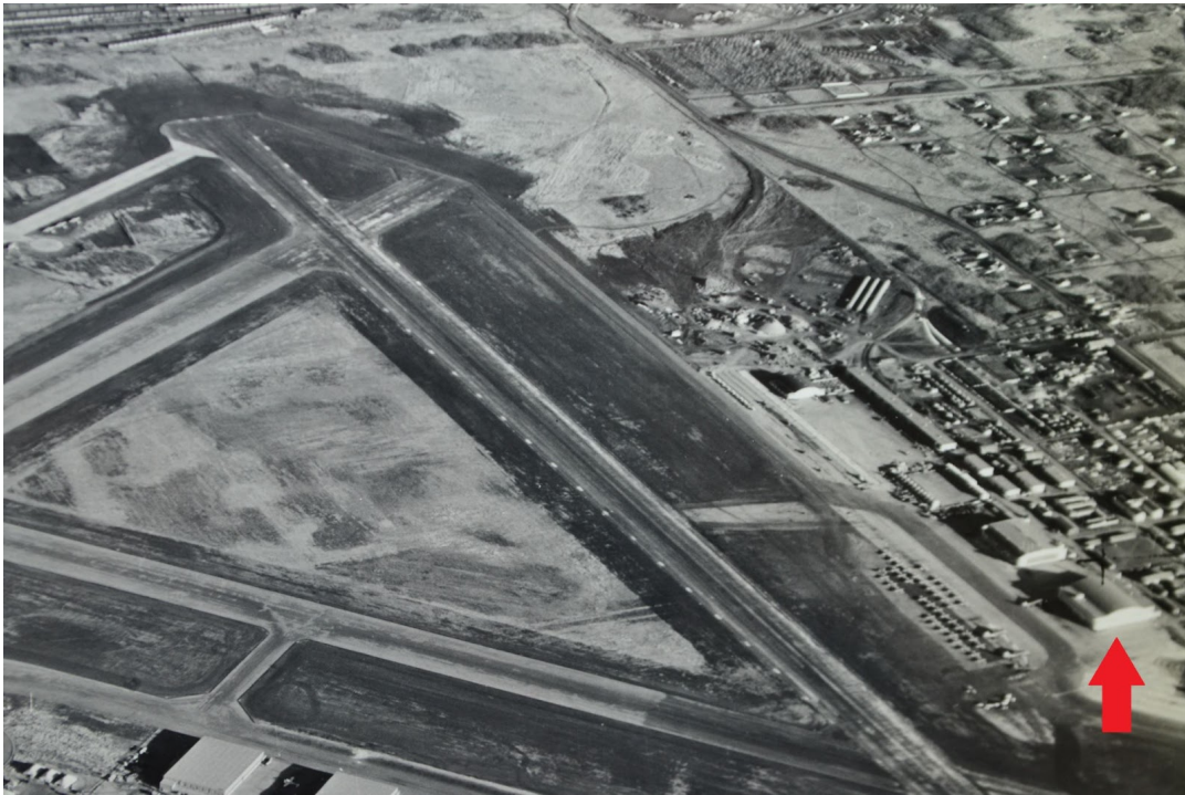
Hangar 11, shown with red arrow, 1943, looking northeast.
