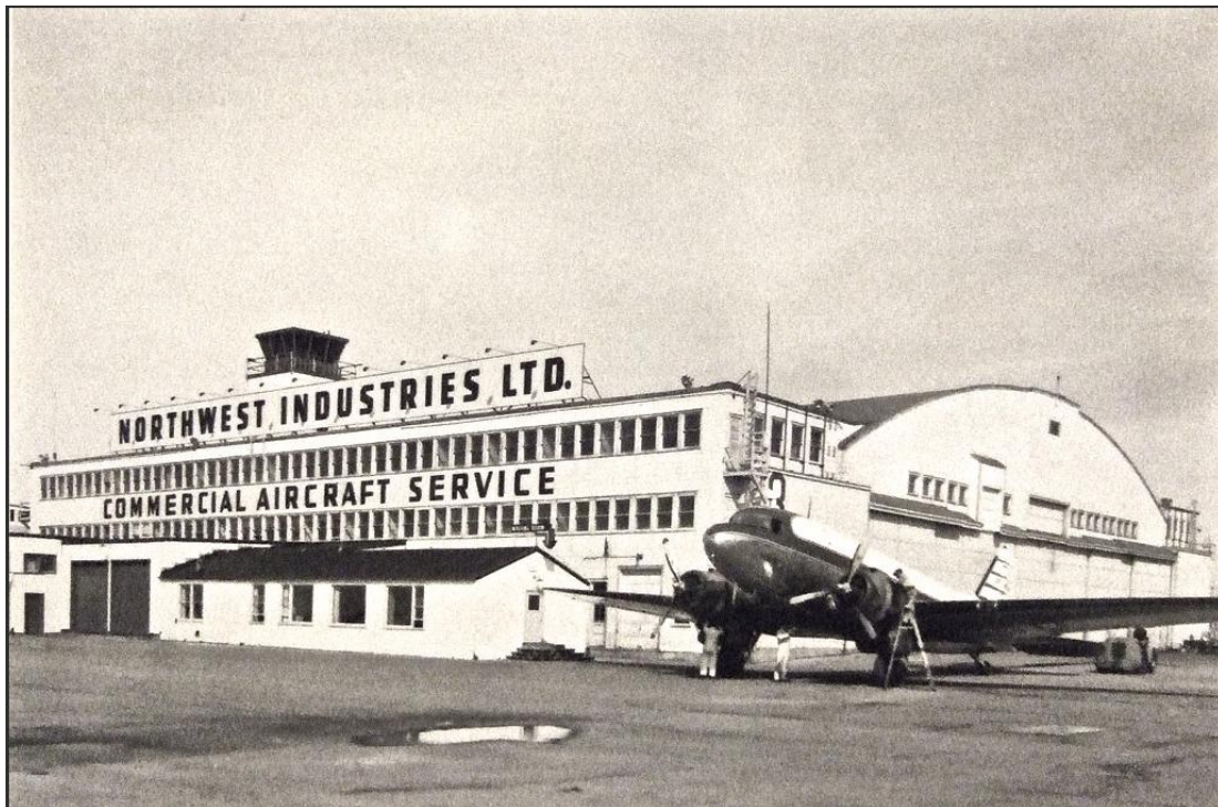
Hangar 11, 1956, looking northeast.
