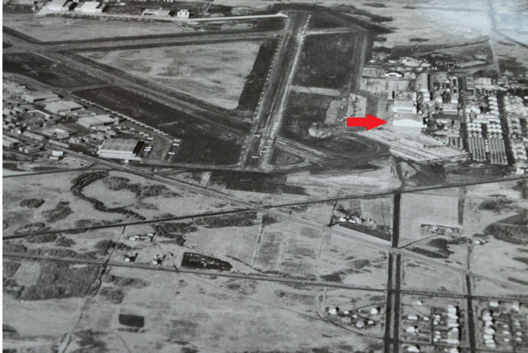
Hangar 11, shown with red arrow, in late 1942 or early 1943, looking north.
