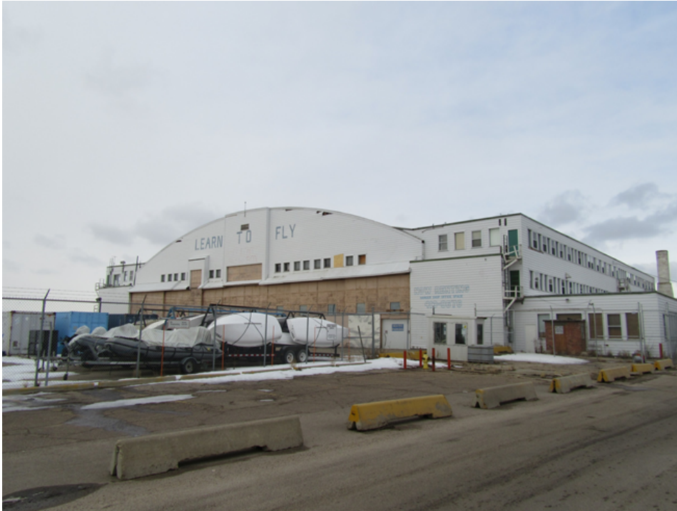
Hangar 11, south and east elevations, looking northwest from 109 Street.
