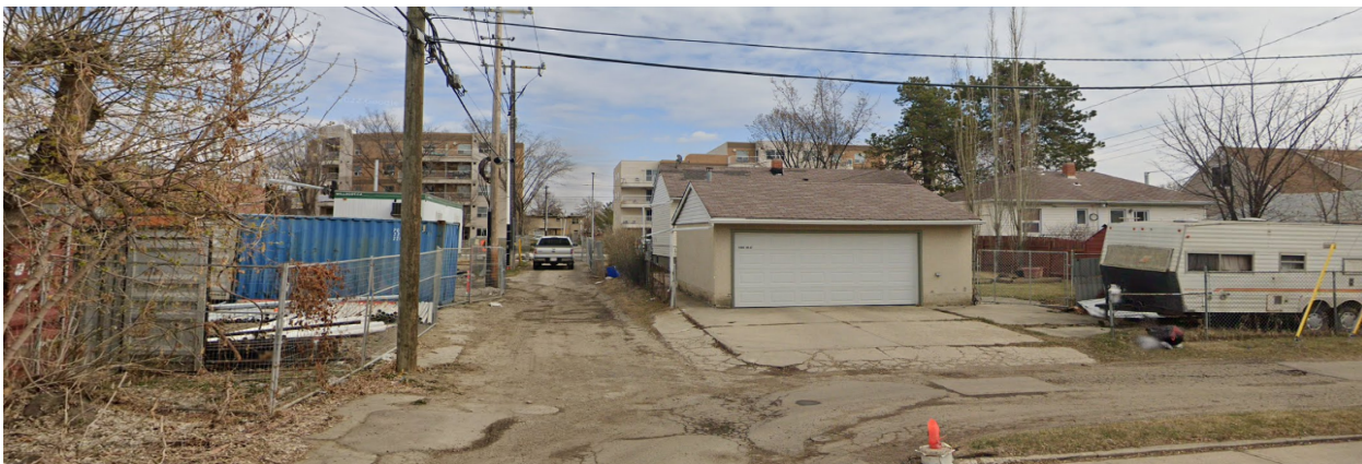
View of the site looking east from the intersection of the adjacent lanes
