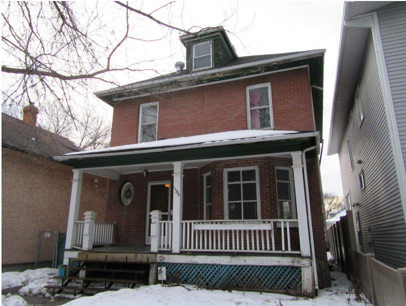
2017, east (front) elevation viewed from 95A Street
