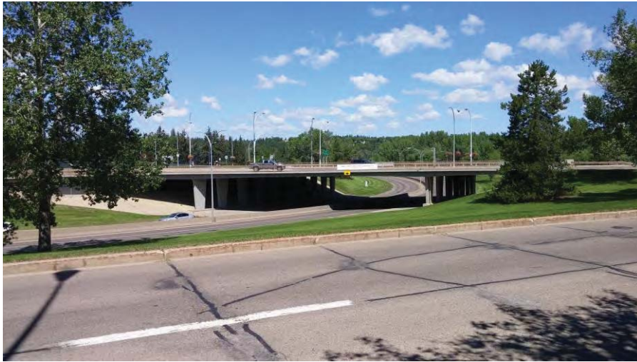
Plate 1.3. Emily Murphy Bridge – view to north (20 June 2016)
