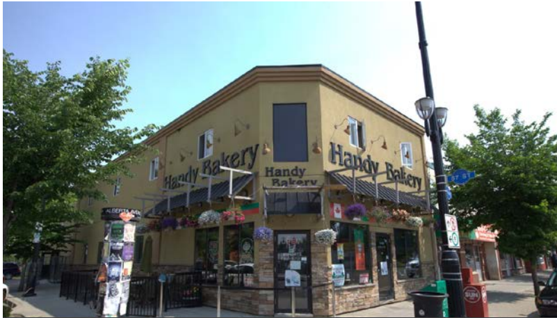
FACADE IMPROVEMENT PROGRAM
