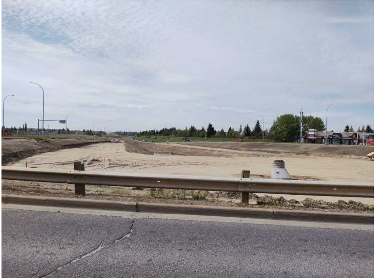
Figure 7. Construction area along Terwillegar Road, south of the project footprint, where vegetation cover had been removed. No obvious bedding could be observed, and the sediments appeared to be reworked.
