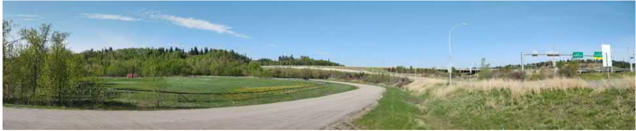
Figure 2. View of Whitemud Drive, looking west, from Fox Drive (on the right hand side of the picture). Note relatively shallow, graded slopes and heavy vegetation cover.
