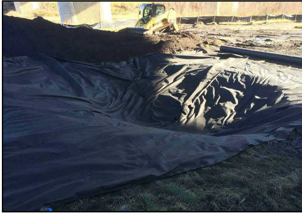
Photograph 7: A seepage pit was re-constructed with a non-woven geotextile liner beneath the drainage culvert on the Whitemud Drive overpass (October 21, 2016).
