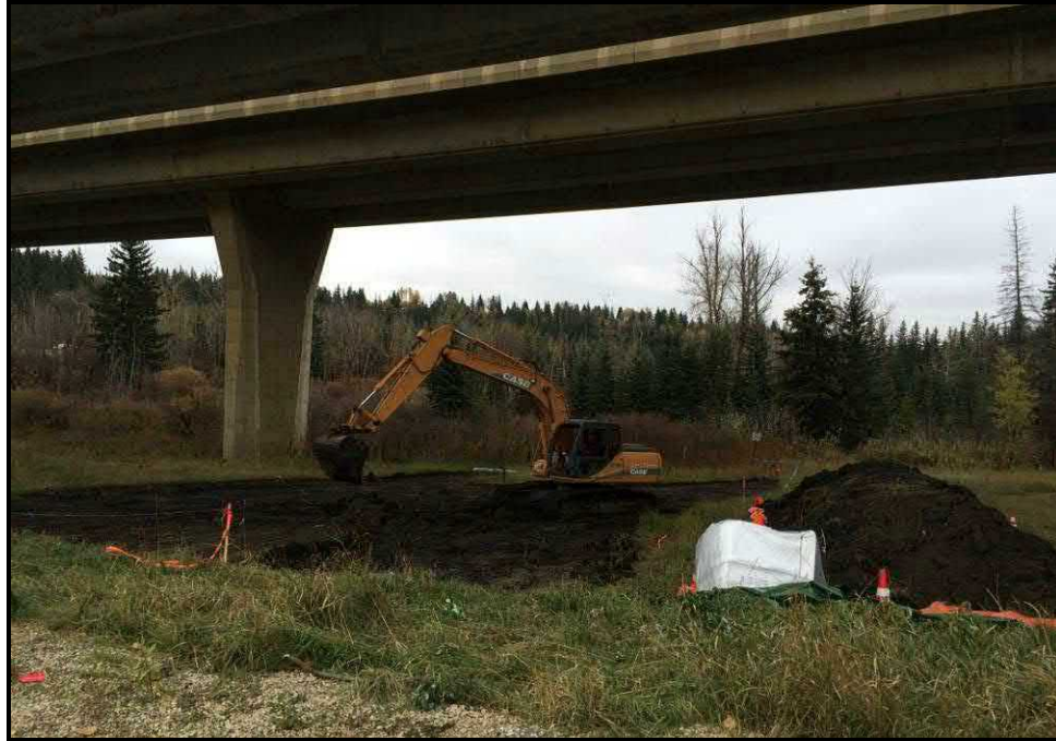
Photograph 3: Excavation of impacted soils from the Site (October 7, 2016).
