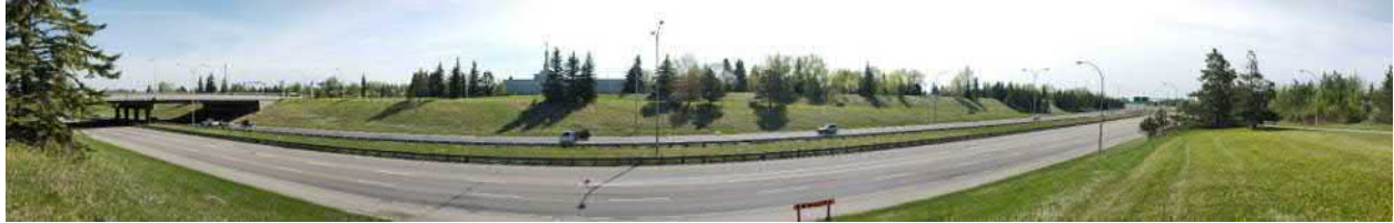
Figure 4. Panoramic view of Whitemud Drive, looking east. The overpass for 53 Ave can be seen on the left hand side of the image. Note heavily landscaped slopes and vegetation cover (erosion control measures) along the entirety of the freeway.
