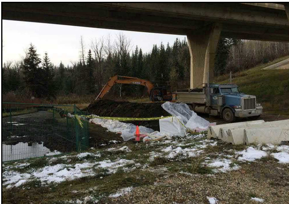
Photograph 6: The impacted soils were removed using tandem gravel trucks, and were hauled to the MCL Waste Systems Class II landfill near Leduc, Alberta (October 13, 2016).
