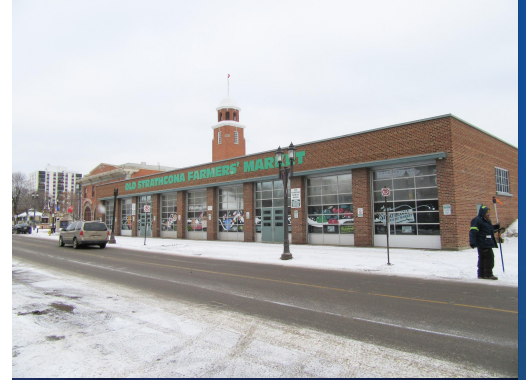
STRATHCONA BUS GARAGE
