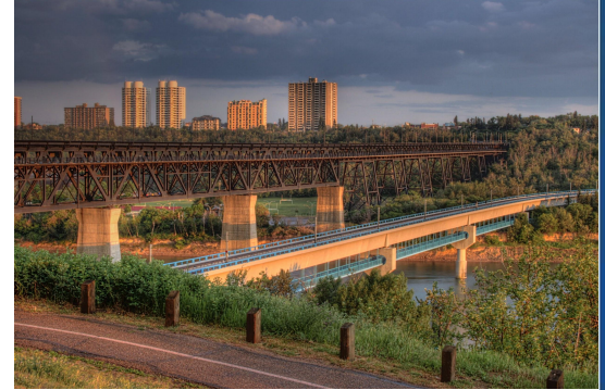
HIGH LEVEL BRIDGE
