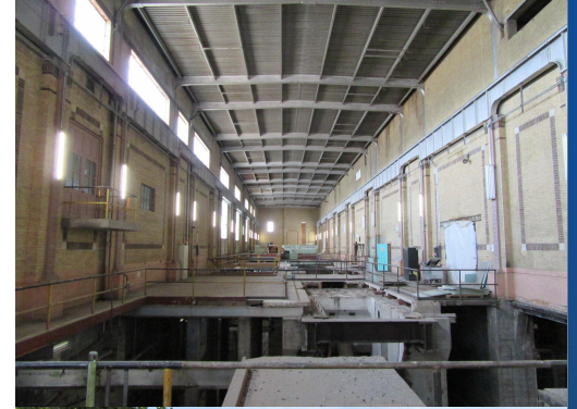
ROSSDALE POWER PLANT
