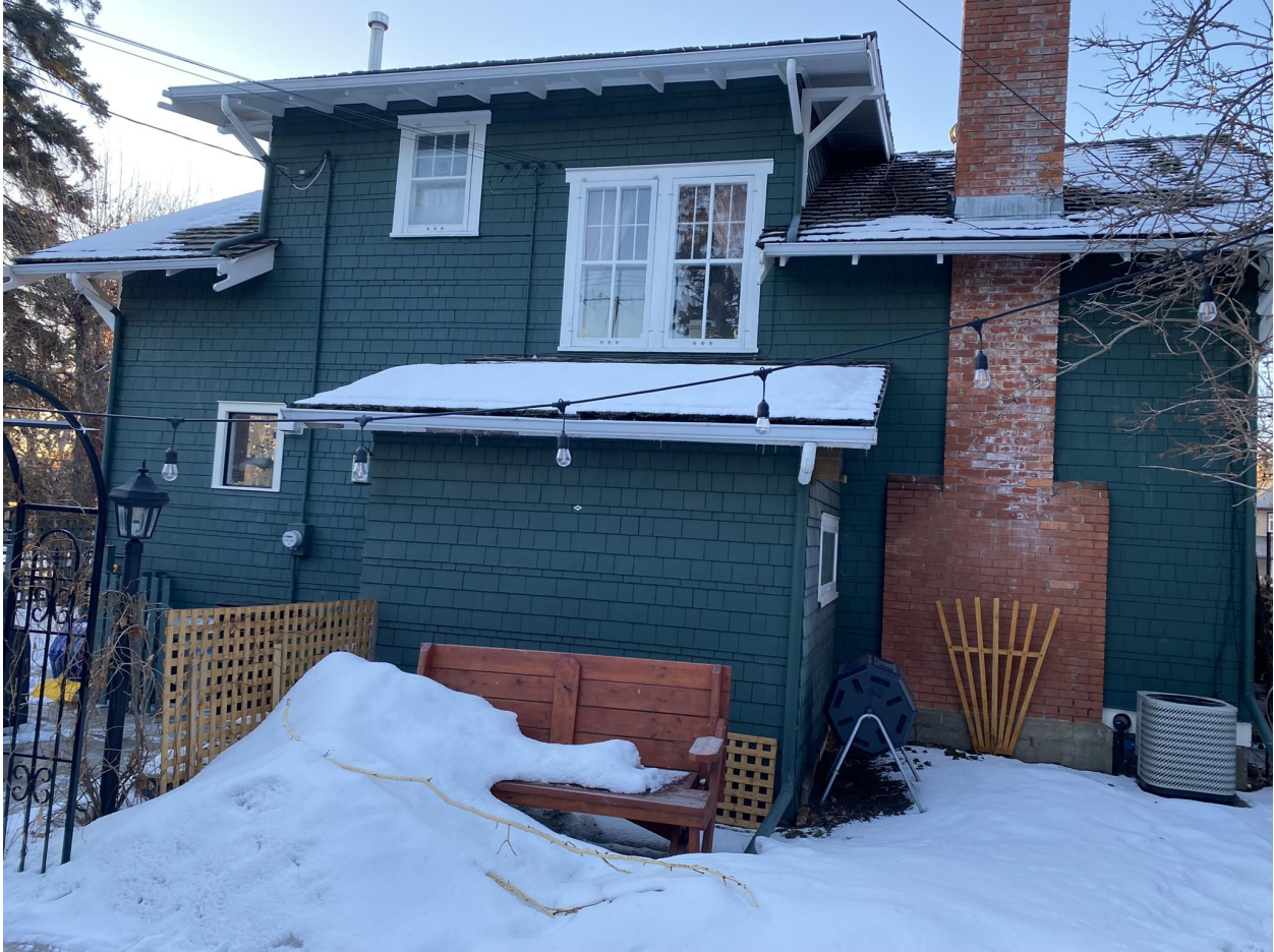
North (rear) elevation, looking south from property rear yard.
