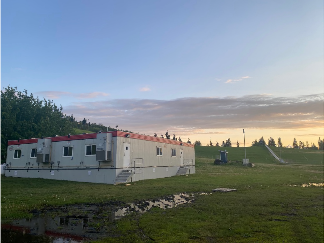
48x60' Modular Facility Installed by Edmonton Folk Festival under Special Event Permit
