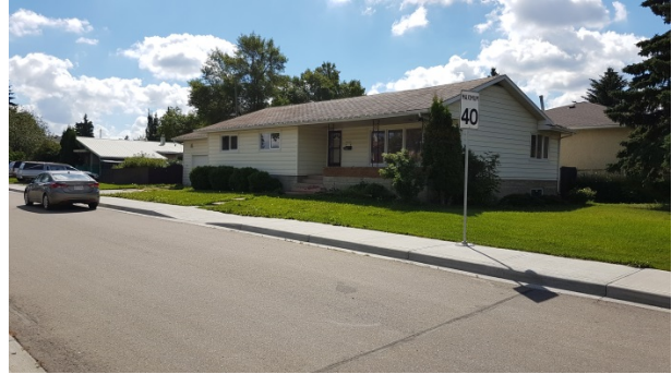
VIEW OF THE PROPERTY, FACING SOUTHEAST
