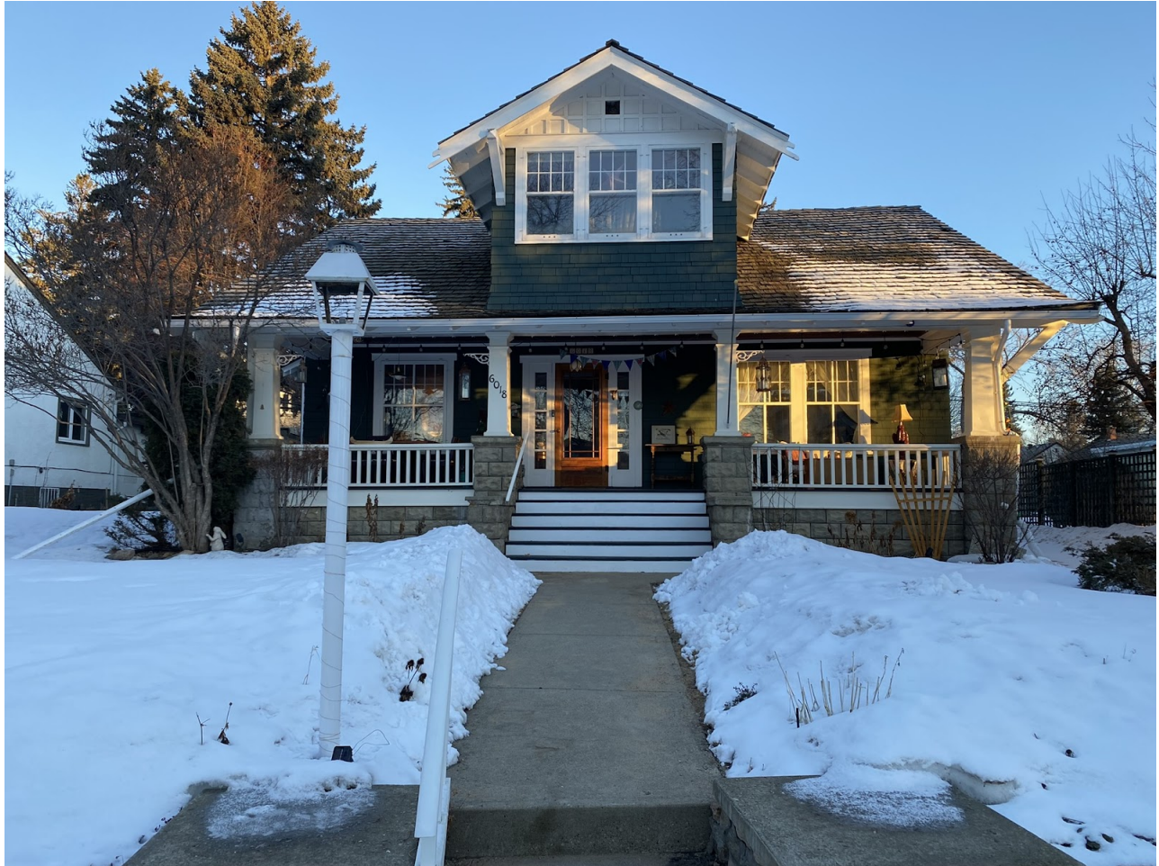
South (front) elevation, looking north from 111 Avenue NW.
