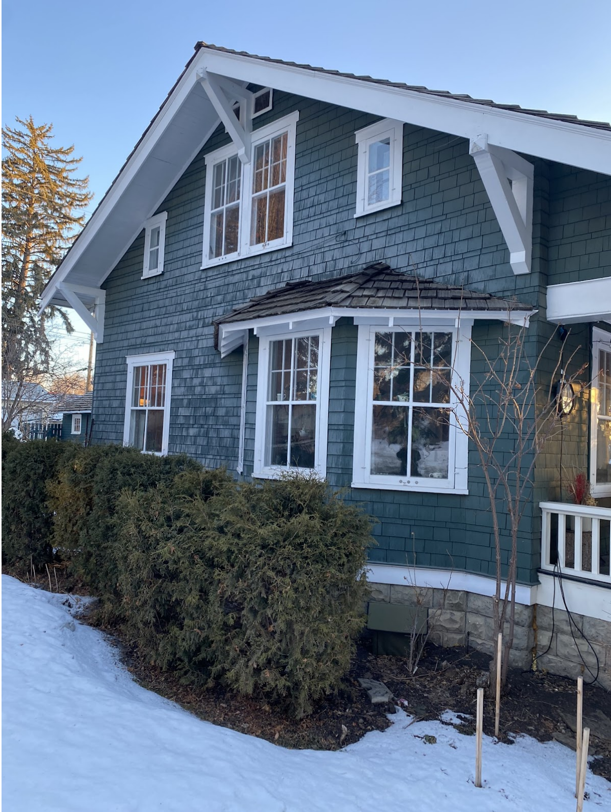
West elevation, looking northeast.
